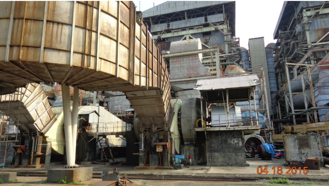
Image 4: Ghorashal Power Station Unit #4
