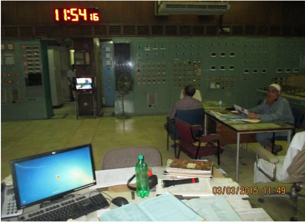
Image 3: Control Room of GPS Unit #4
