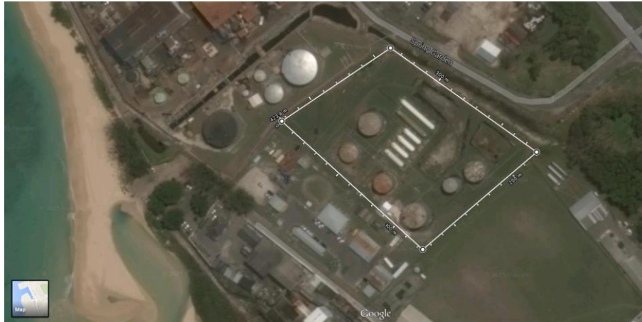
Figure 4: Spring Garden Location of the proposed LNG receiving, storage and re-gasification facility
