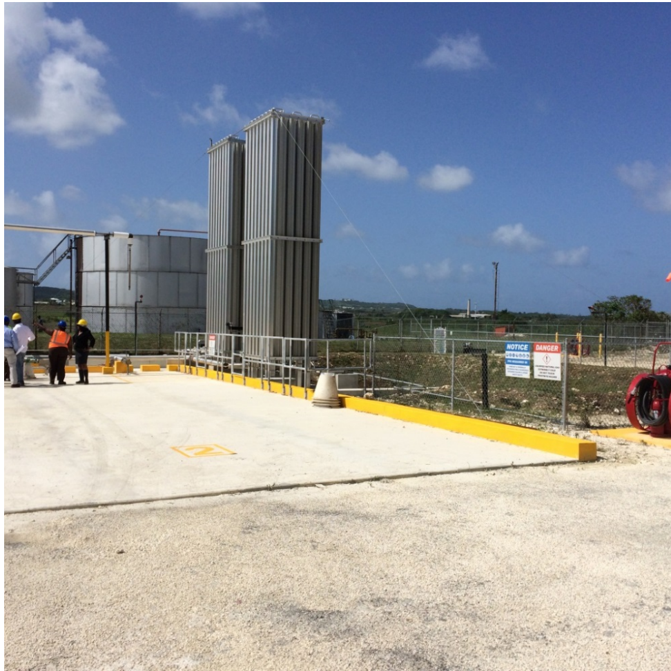
FIGURE 2-3 ISO-CONTAINERS/TANKS UNLOADING PARKING AREA AND VAPORIZERS
