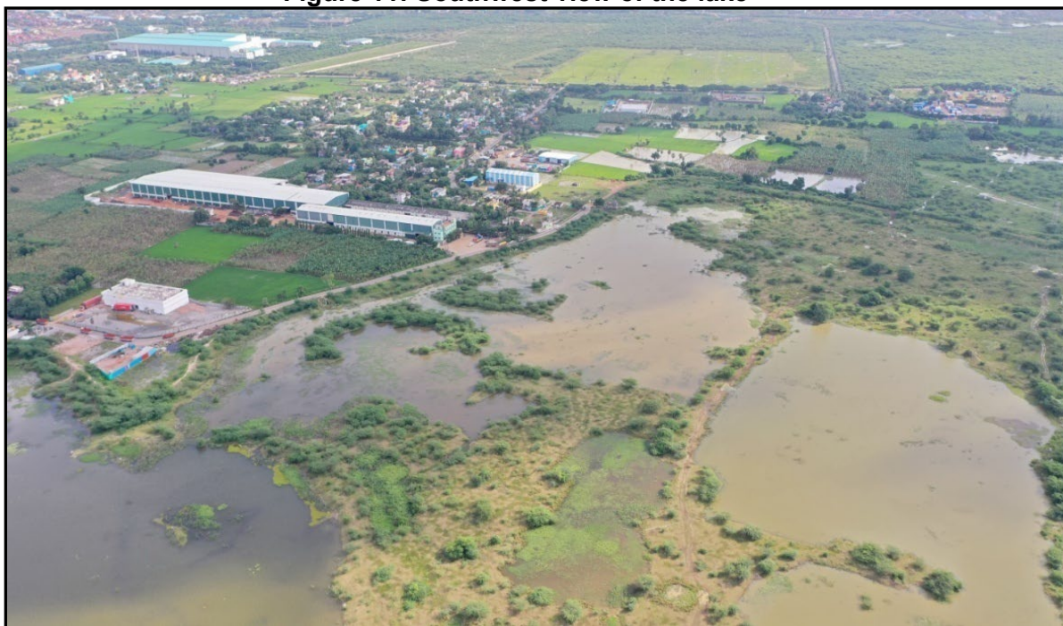
Figure 11: Southwest view of the lake
