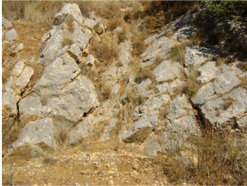
Figure 4.3: Highly Fractured and Jointed Mdairej Limestones on the Right Bank of the Reservoir
