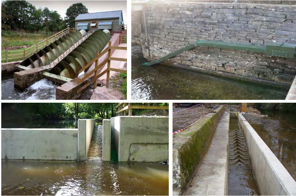
Figure 2. Different types of passes suitable for the freshwater eel (source Internet)
