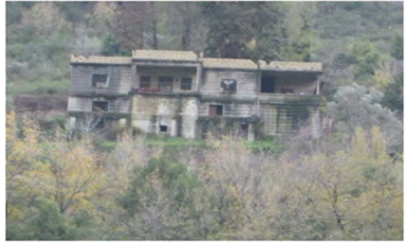
A substantial residence now used by seasonal workers
