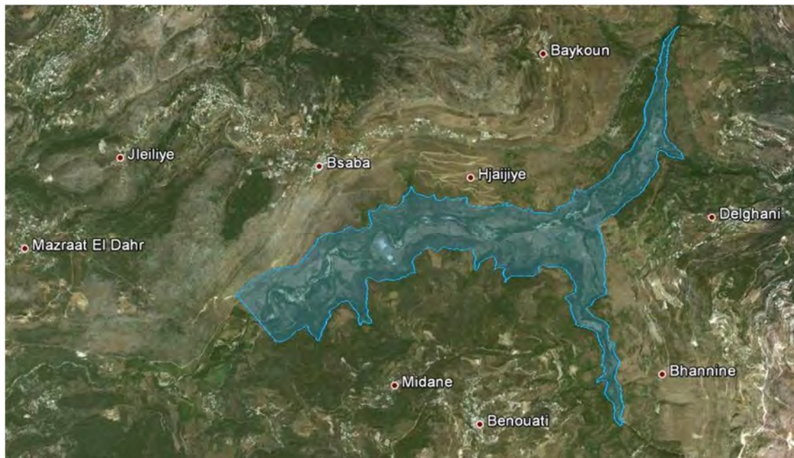
Bisri Dam and Reservoir on Nahr Bisri
