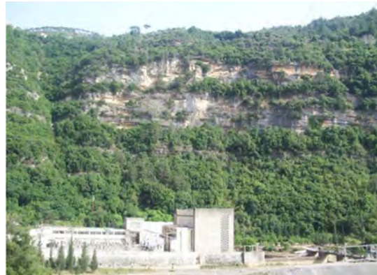
Joun Hydropower Plant
