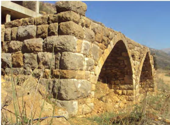
Arches, c.350 m upstream from the church
