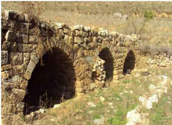
Remains of the monastery stables
