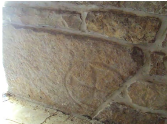
Broken engraved stone indicating the church has been rebuilt
