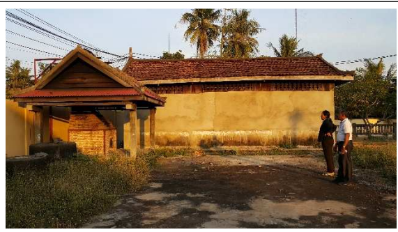
Malfunction incinerator - Kampong Thom RH
