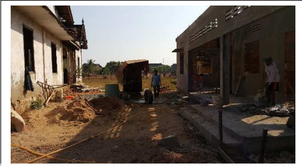
Concrete mixing machine that block passage to Toilet – Sambo HC
