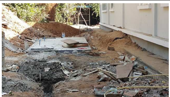
Construction waste – Stoung RH
