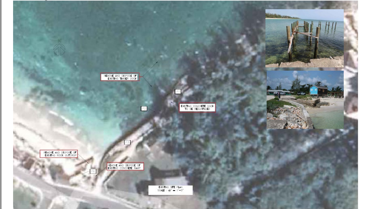
Figure 21. Nicholls Town dock, North Andros, Bahamas. Source: Ministry of Works & Utilities.
