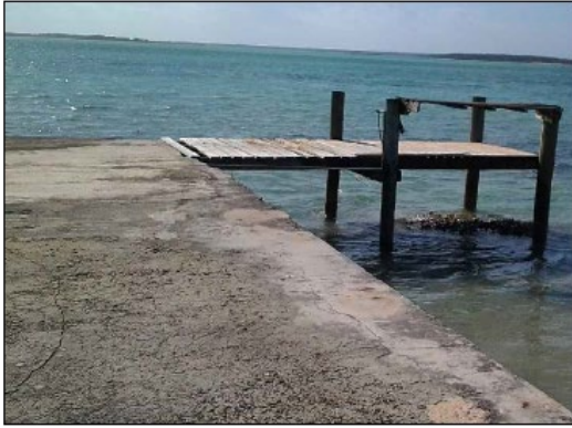
P1 VIEW LOOKING AT PILES NORTH EAST
