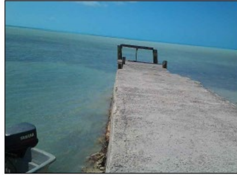
P5 BIRD'S EYE VIEW OF ABUTMENT
