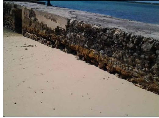
P2 LOOKING SOUTH EAST AT ABUTMENT SIDE
