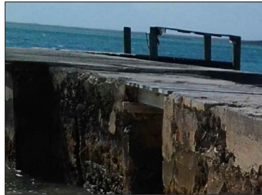
P4 VIEW LOOKING SOUTH EAST
