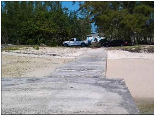
P3 VIEW LOOKING AT ABUTMENT NORTH WEST
