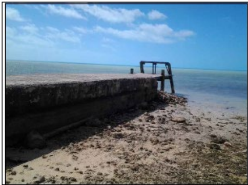
P2 VIEW LOOKING AT ABUTMENT SOUTH WEST
