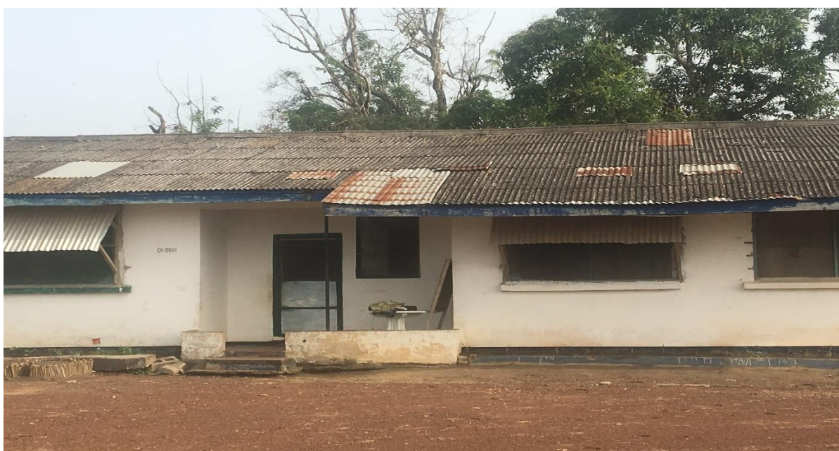
Figure 4 Part of staff house with asbestos roof sheet to be rehabilitated
