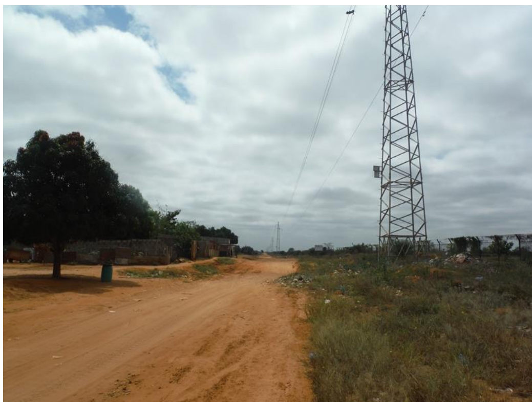
Wmk 510 view north – village of Quenguela Norte to west (left) side, narrowing RoW to 8-10 m.
