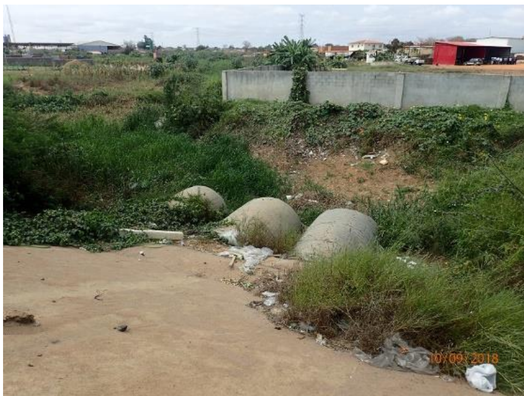
Culvert on the south side of Via Expresso to be used to convey water under the highway. Culvert is 1.3 km east from E.L.P/Via Expresso junction.
