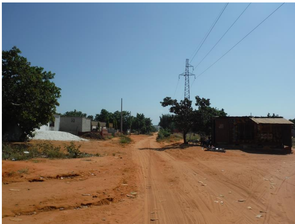
Wmk 523 view west – constraint of property to south and MV powerline to north
