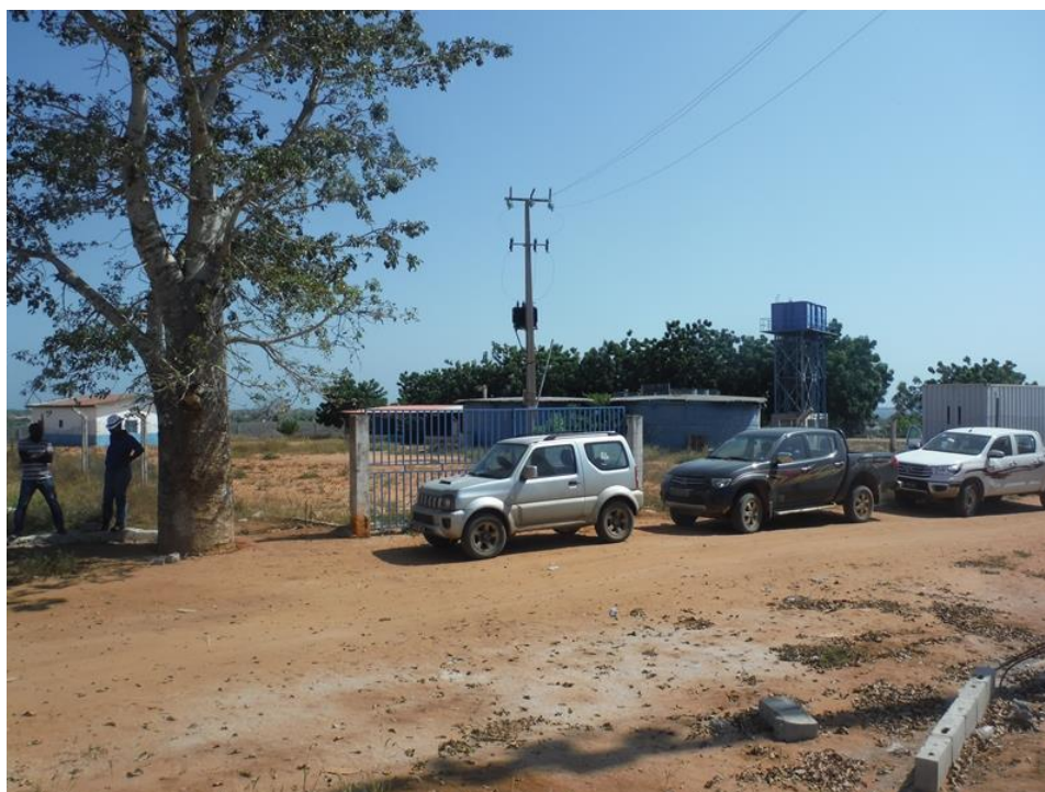
Corner into CD Ramiros – view west into proposed site
