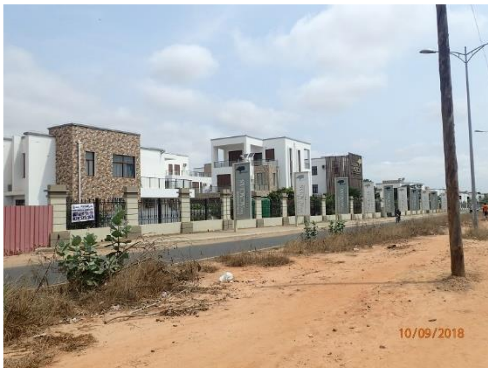
Portuguese residential area on left (west) side of alignment approximately 0.5 km north of crossing point.
