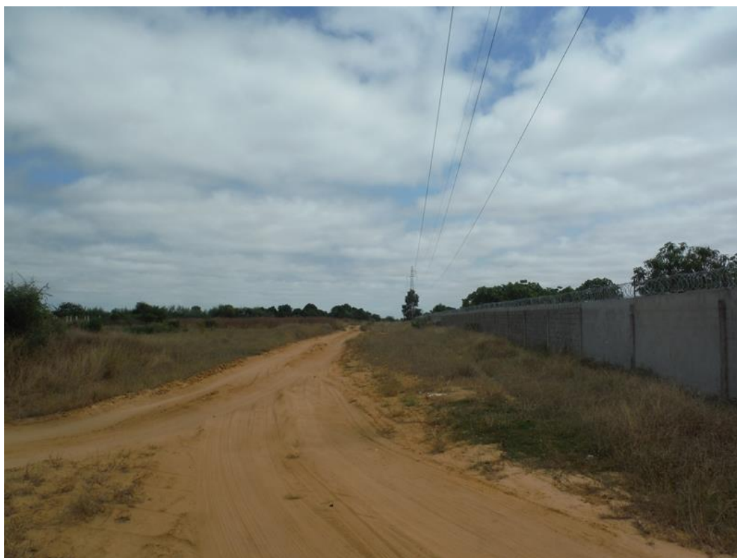
Wmk 508 (Node 1) view west with wall and MV powerline to the north (right) side
