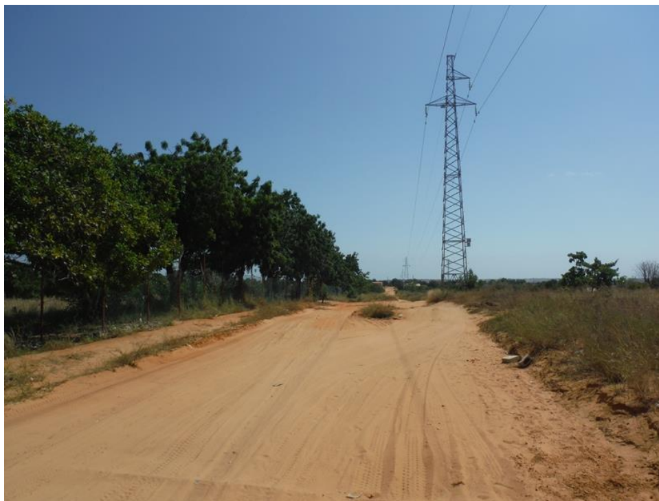
Wmk 522 view west – constraint of property to south and MV powerline to north
