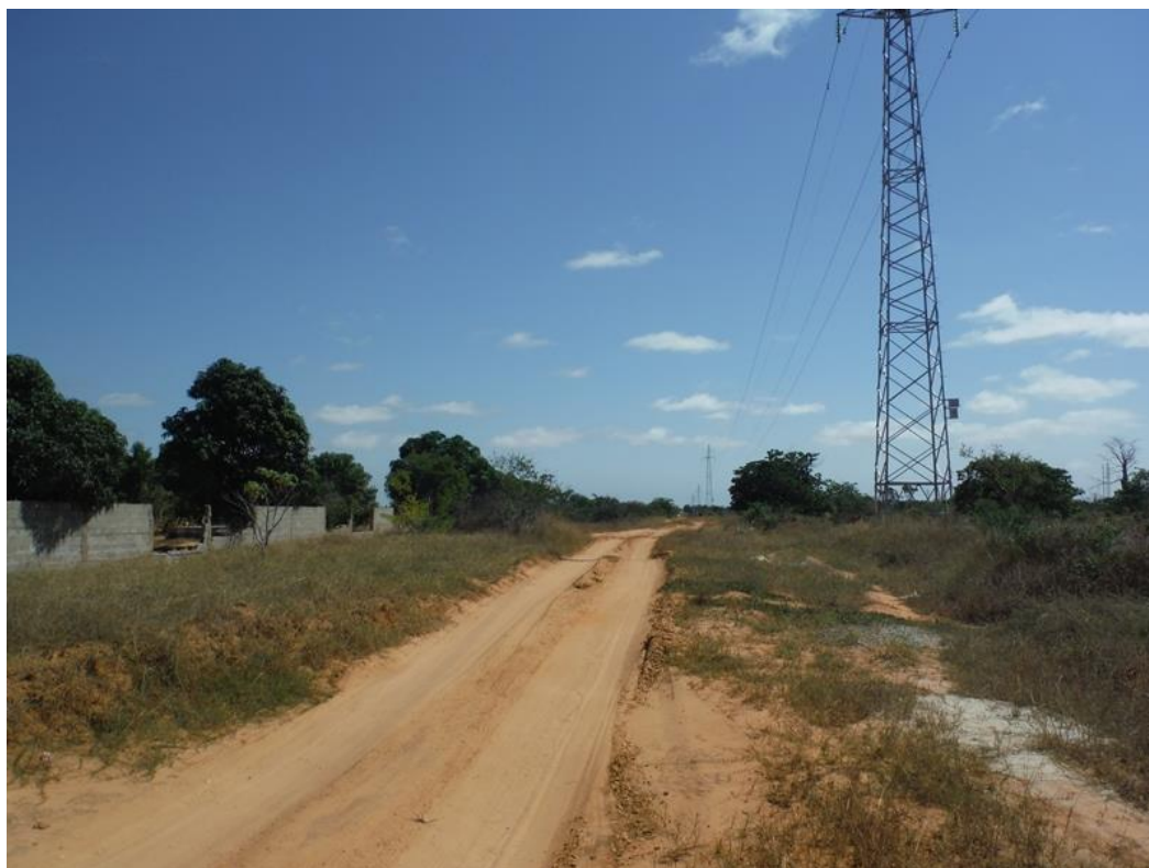
Wmk 516 view west – walled property to south side and MV powerline to north side
