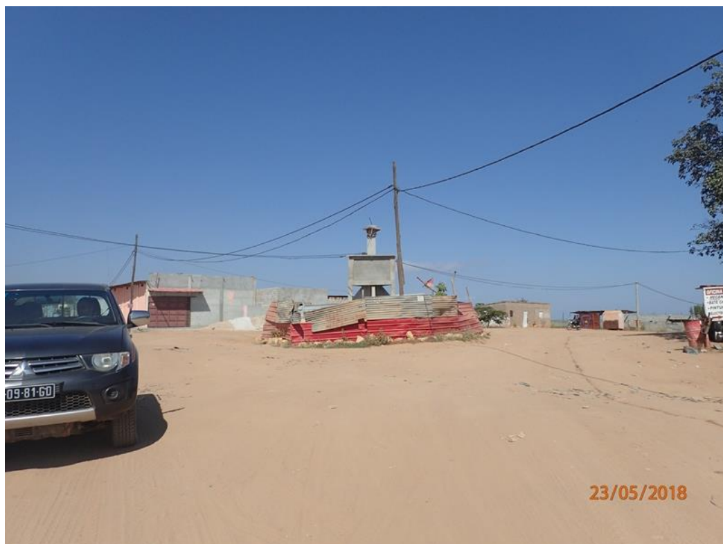
View north from Wmk 525 towards roundabout – pipeline alignment turns to north-west
