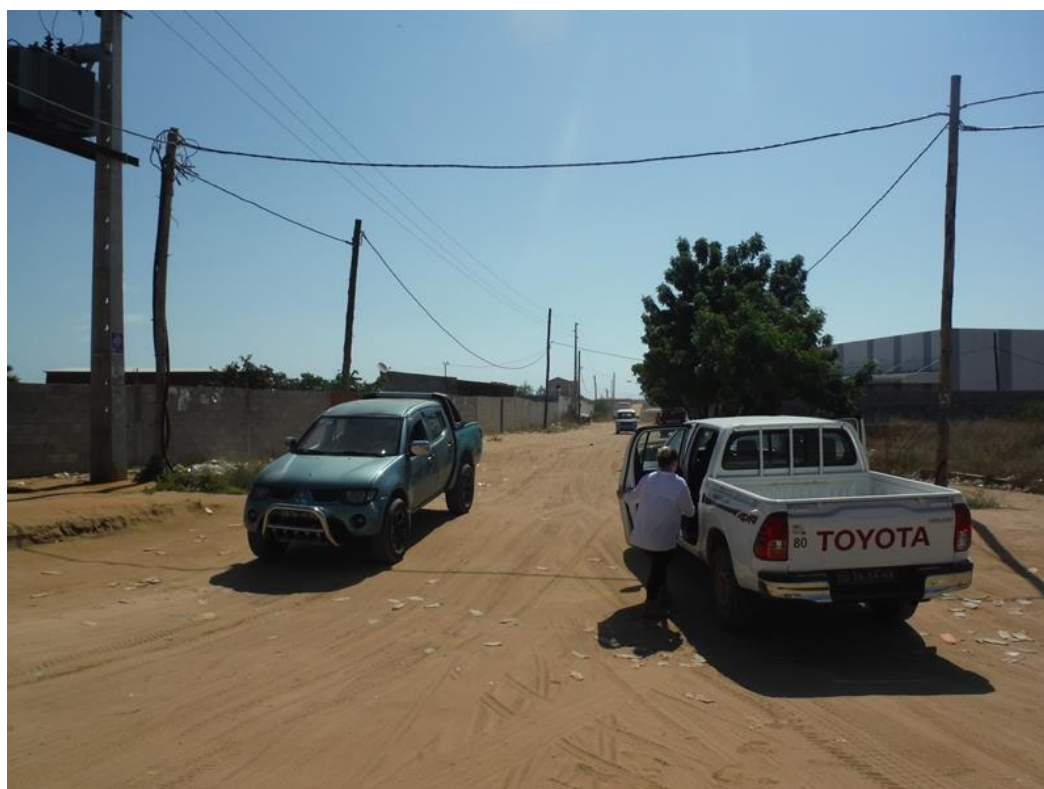
North-west towards CD Mundial - wider track (10-12 m) with LV powerline constraints
