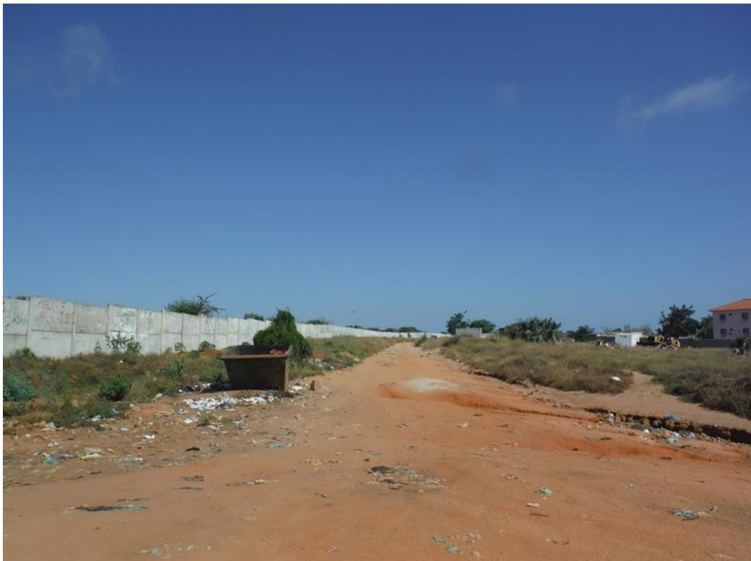
Wmk 530 view south from corner in direction of pipeline alignment
