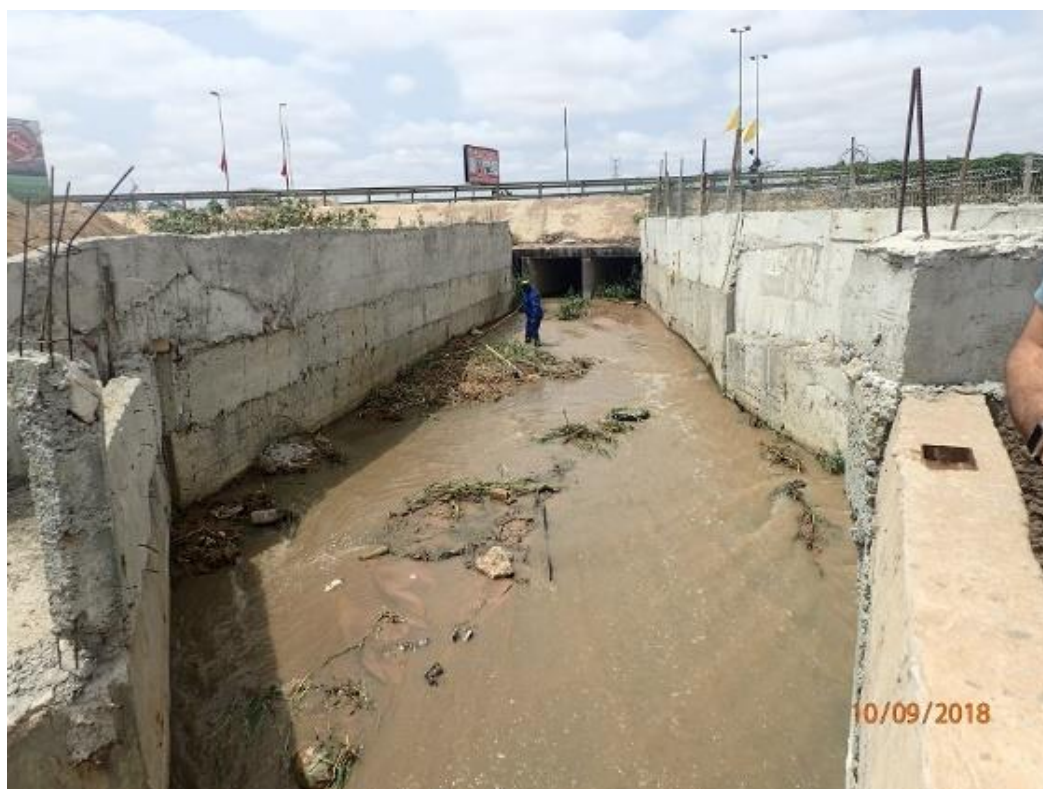
Culvert from northern side of Via Expresso looking south.
