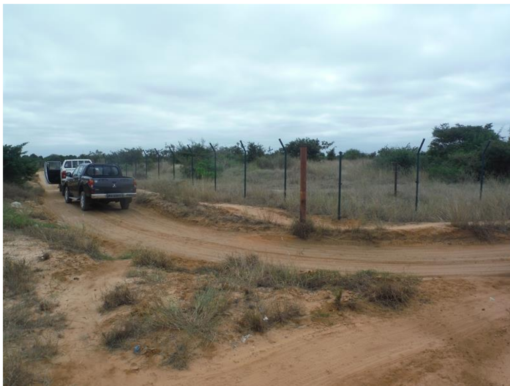
Wmk 503 where transmission pipeline turns north towards Quenguela village
