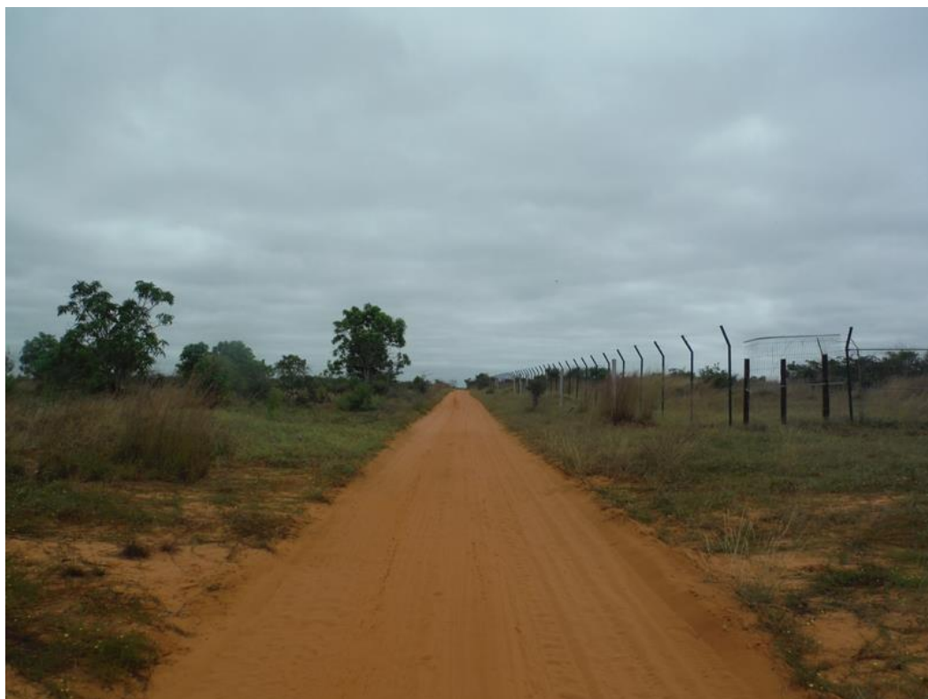
Boundary fence to north (right) side of track – extending for 4 km
