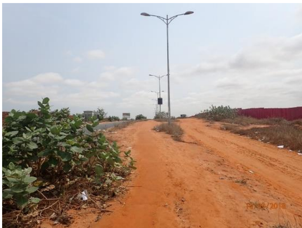
Alignment 0.2 km north of roundabout (1.2 km north of crossing point) – view north.
