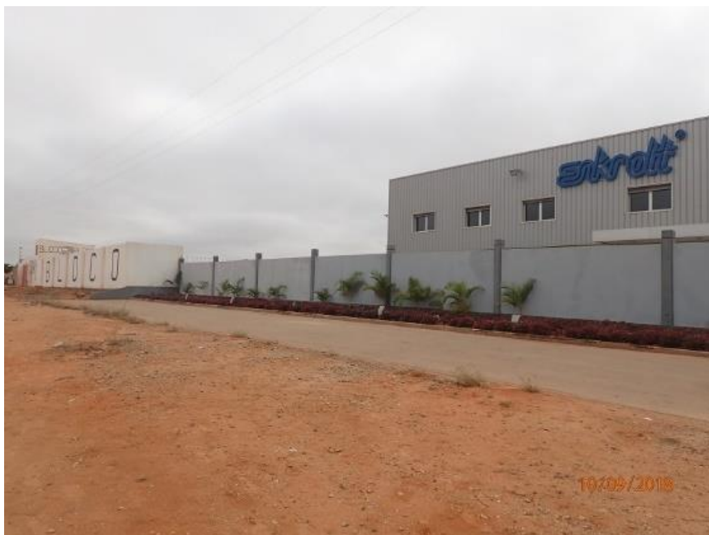
Industrial buildings on the right (east) side of the approximately 3 km from Node 2.
