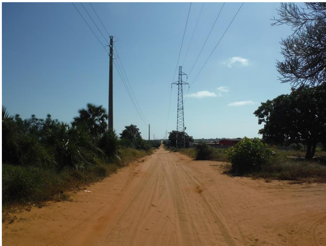
Wmk 528 view west – space between powerlines (left and right) narrows to 4-6 m
