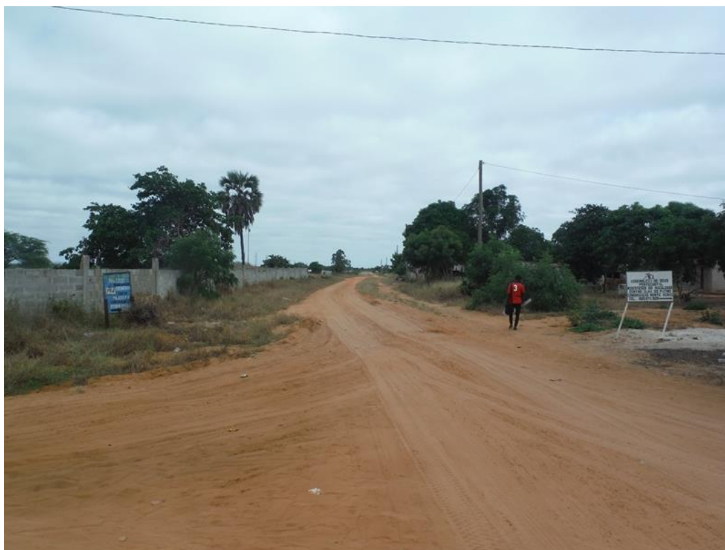
From Wmk 506 (Quenguela village) view west along pipeline route and Estrada Lar Patriota
