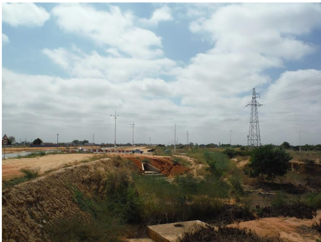
Wmk 513 – view north-east across eroded hole with storm drain in base to be crossed
