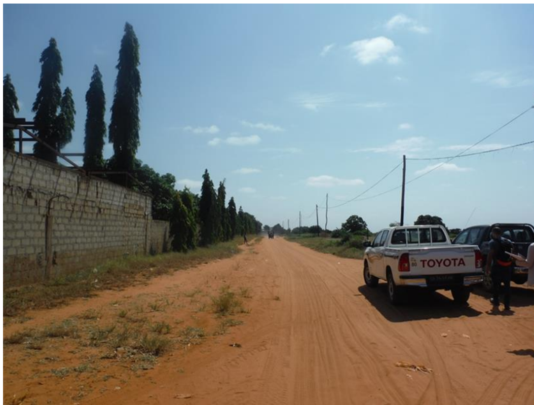
View north along pipe alignment out of WTP and CD Bitu – note power line to the east (right)
