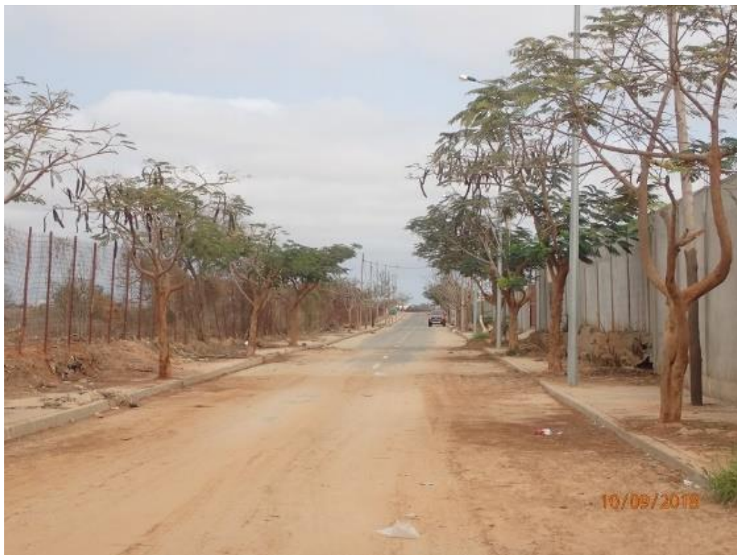
Example of asphalted side road 3 km along the alignment looking west.
