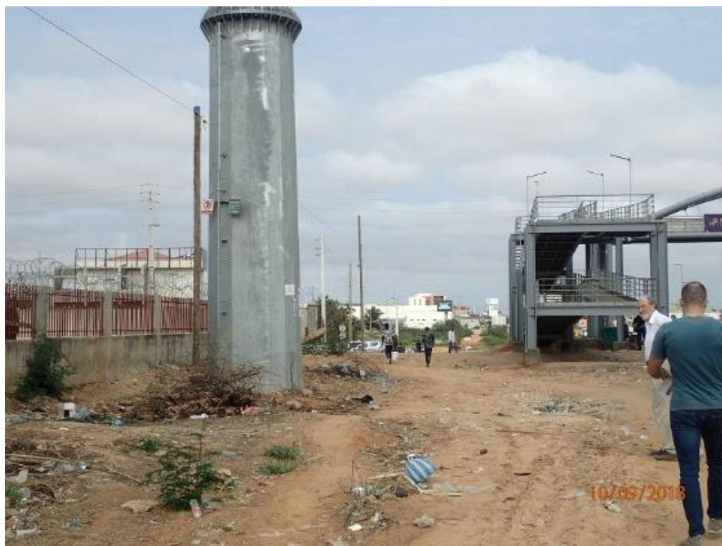
Pinch point between power pylon and the foundations of pedestrian footbridge over the Via Expresso- view westward of junction between E.L.P and Via Expresso.
