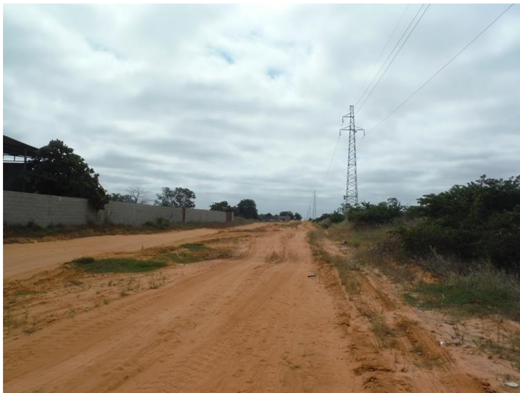
Wmk 509 view north – 15 m between property wall to west (left) and powerline to east (right)
