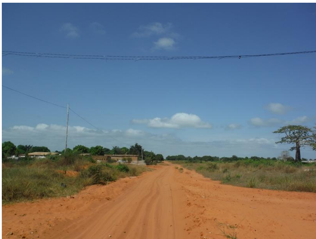
Wmk 481 at Bitá WTP crossroads - view south – properties on left (east) side, clear land to right (west side)
