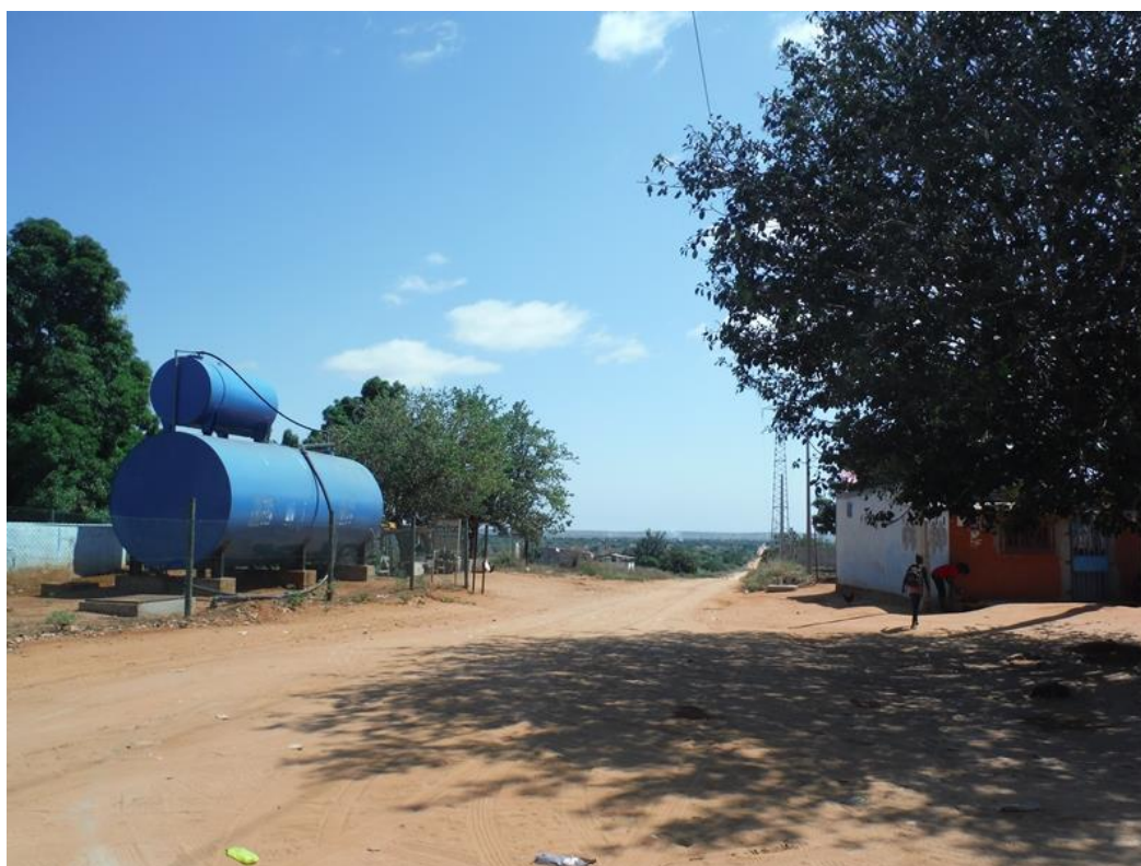
Wmk 520 view west – within Tanque Serra village with property and powerline constraint on north (right) side and water tank and concrete reservoir on south (left) side
