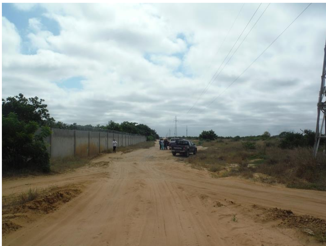
Node 1 at Wmk 508 – looking north
