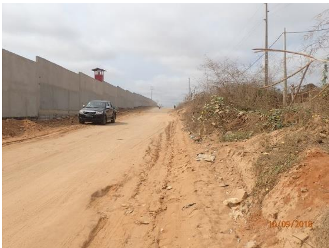
Concrete wall marking the border of a significant 82 ha compound on the right (east) side of the track-view south-east toward Node 2.
