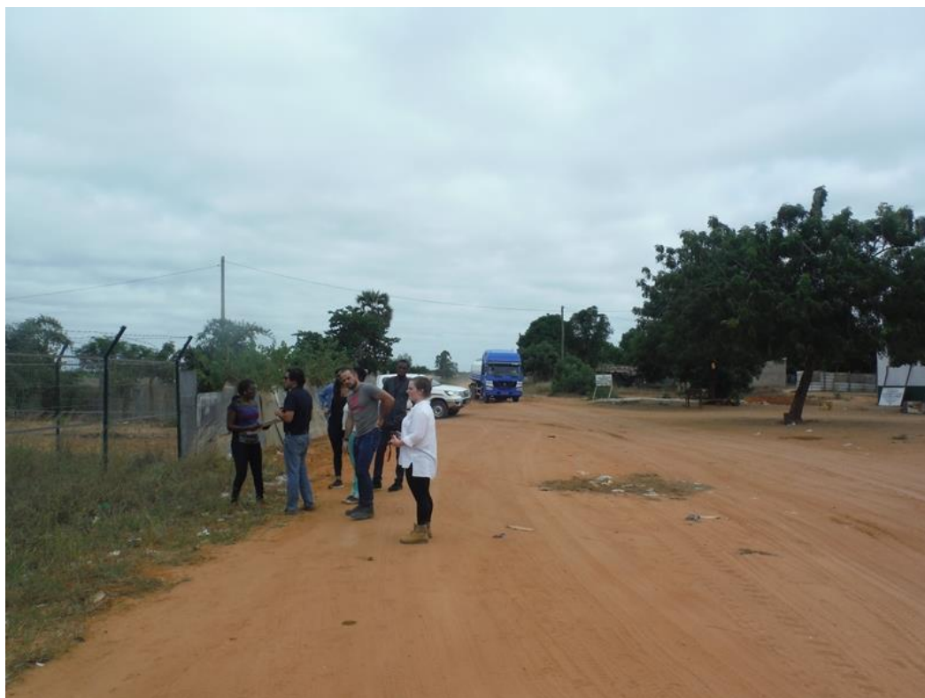
Wmk 506 - the point where the transmission pipeline (from the left) meets Estrada Lar Patriota
