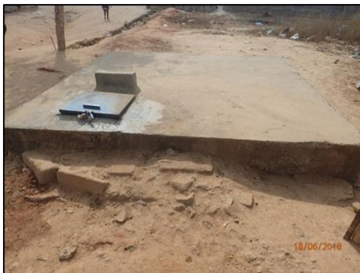
Plate 6-8: Privately-owned underground water tank in Mundial service area.
