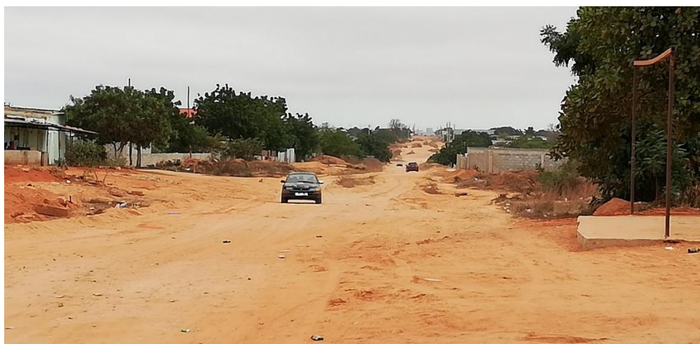
Plate 2-20: The Pipe Alignment from CD Cabolombo to Via Espresso
