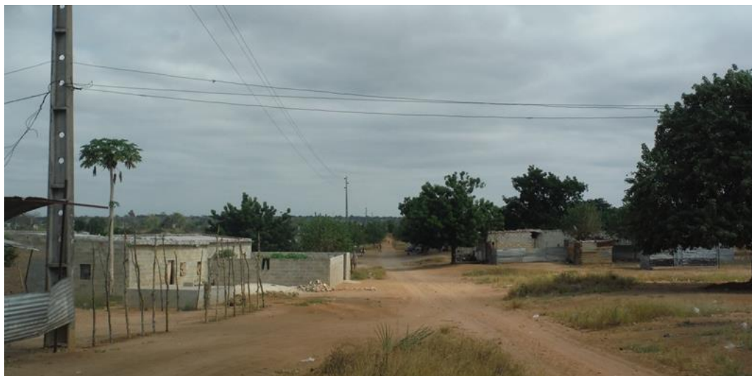
Plate 2-4: Pipeline Route through Julio Village.
