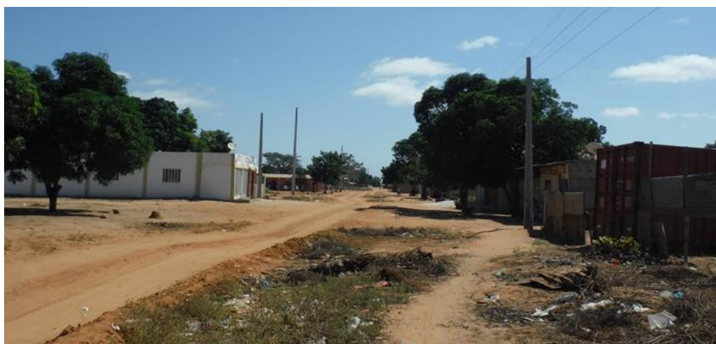
Plate 2-24: The eastern entrance to Tanque Serra village.
