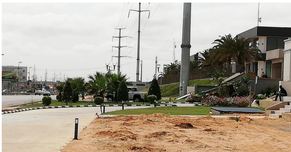
Plate 2-23: The pipeline will cross the entrances to several large premises
