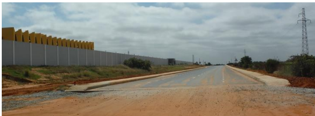
Plate 2-18: The start of the asphalted road that will continue to Via Expresso .
