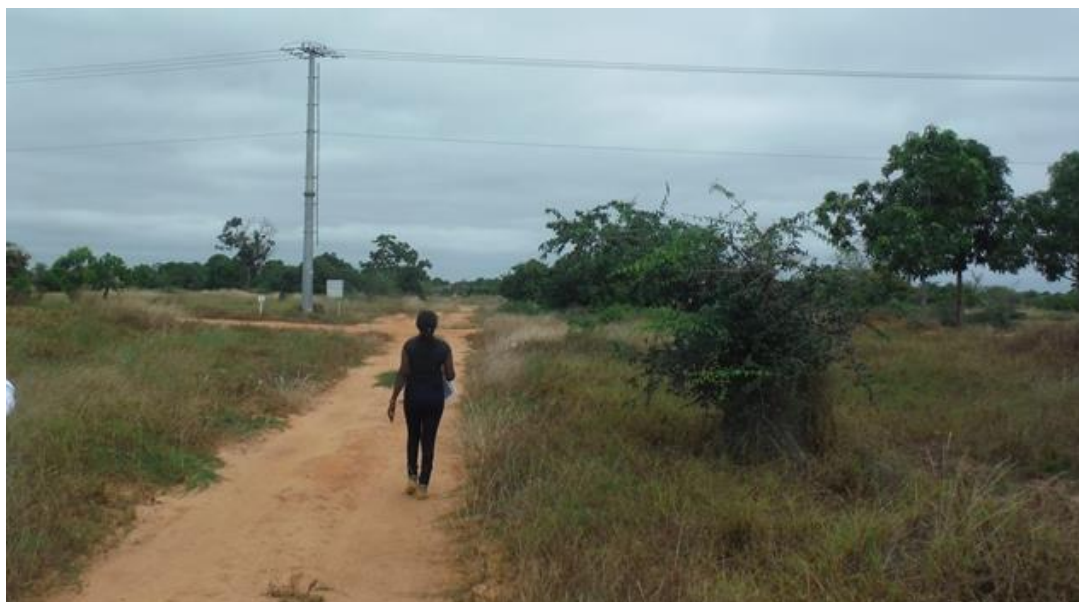
Plate 2-10: A MV power line and buried water line crossed by the B4WSP alignment.
