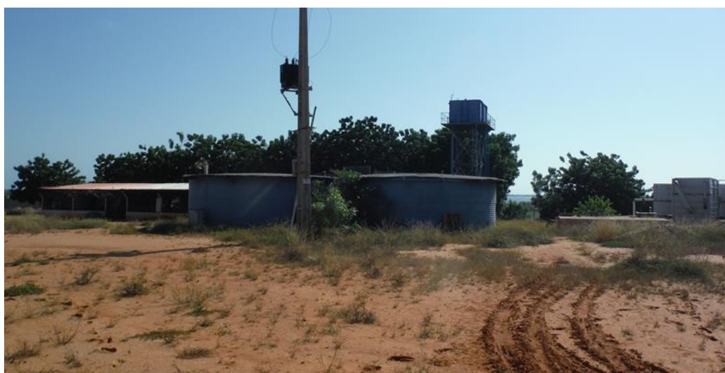
Plate 2-35: CD Ramiros, previously a local distribution centre.
