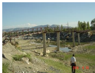
Pedestrian bridge over Akburasai
