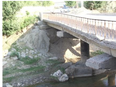
Bank protection site over Namangansai
