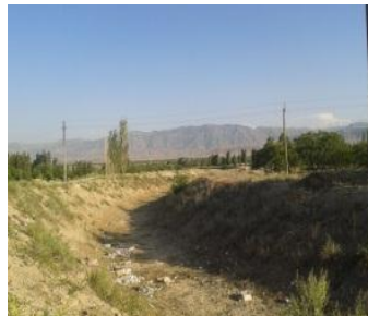
Mudflow canal in southern border of Kaptarhona settlement
