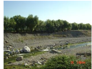
Collapse of bank in Akburasai
