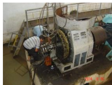
Repair works at Orom PS (Istiklol)
