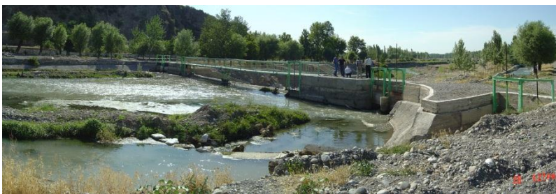
Structures (Kambarata hydrosystem). Water intake into Beshtol, Robdon, Yangi canals
