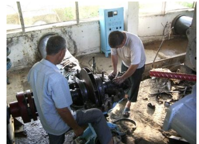
Repair works at PS Urikzor
