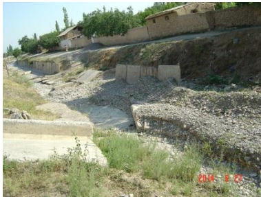
Bank protection site over Namangansai
