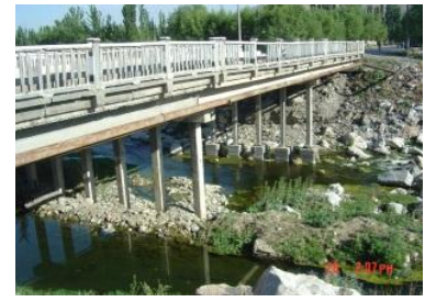
Road bridge over Akburasai
