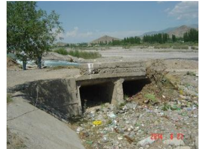
Inverted siphon damaged by mudflow
