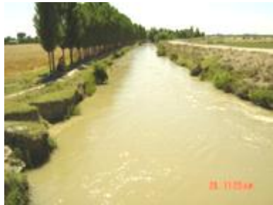
Bank erosion in Savai canal
