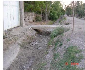
Canal Arabtepasai dry. Water intake into canal in Kyrgyz Republic territory
