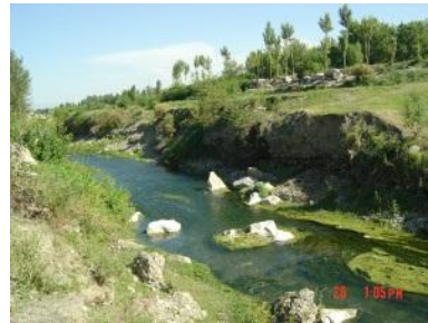
Collapse of bank in Akburasai
