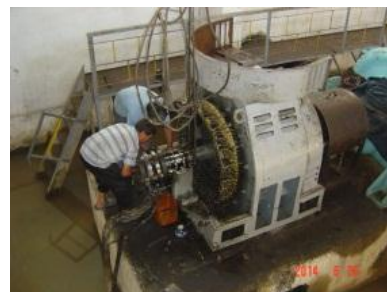
Repair works at Orom PS (Istiklol)
