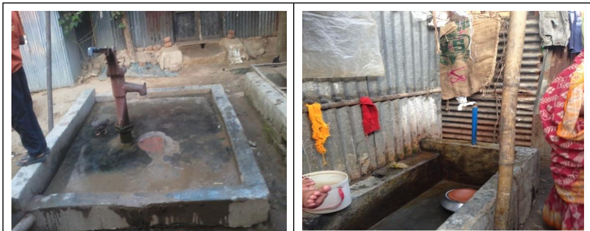
Figure 4.5 Tube-well and pipe water supply at Tikkarchar
