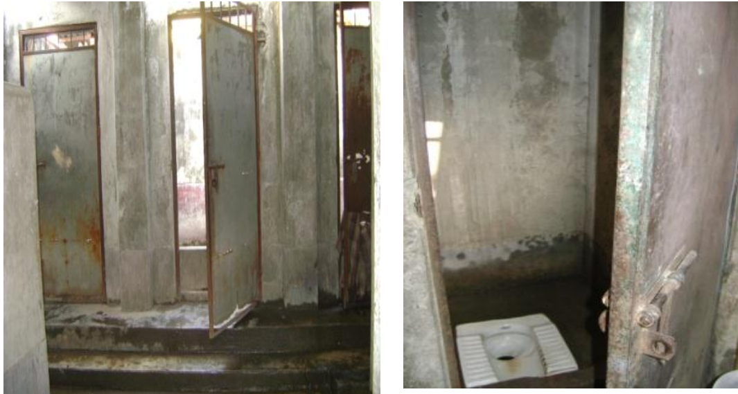
Figure: Sanitation facilities at Rishipara
