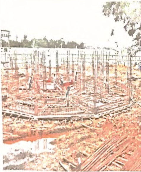
No more dry taps: An overhead tank being built at Mattuthavani in Madurai under the Mullaperiyar drinking water project. • G. MOORTHY
