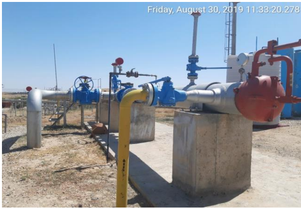
Amine Plant machinery
