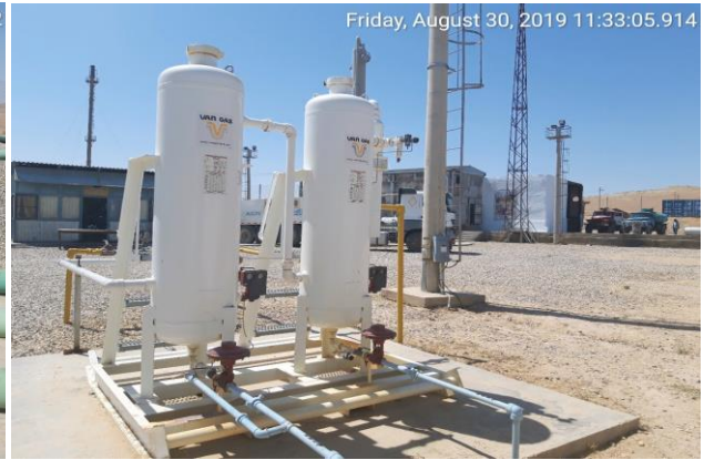
Amine Plant machinery
