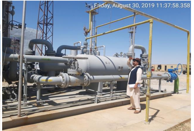
Amine Plant (Sulfur separation)
