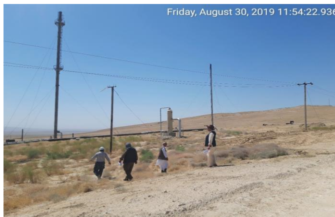
Air pollution prevention system (H 2 S combustion)
