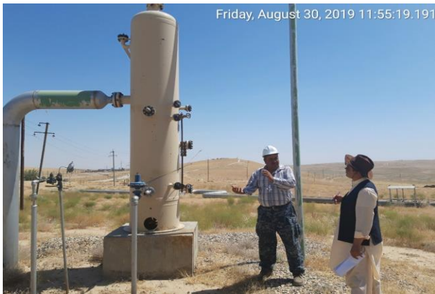
Air pollution prevention system
