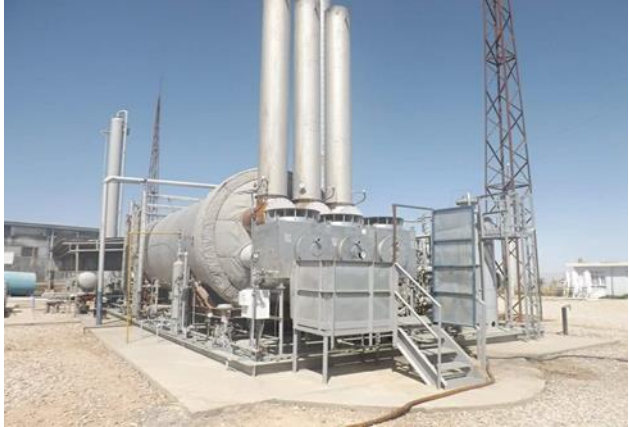
Amine Plant (Sulfur separation)
