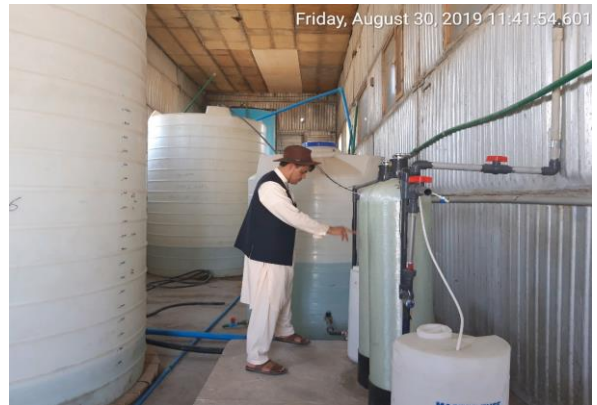
Water purification system for gas production
