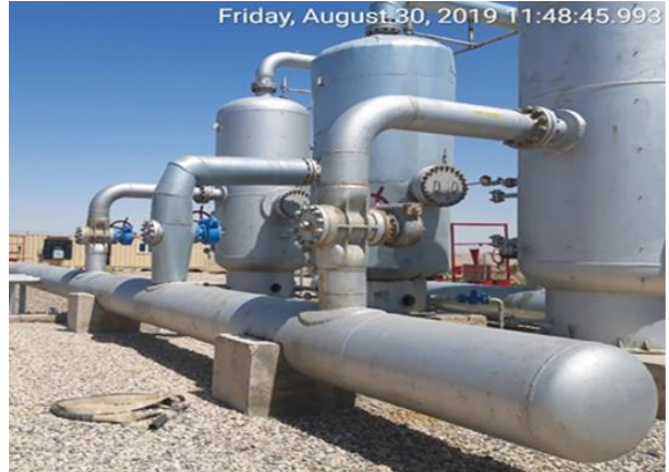
Amine Plant (Gas purification system)
