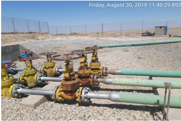
Amine plant (Gas inter to the system)
