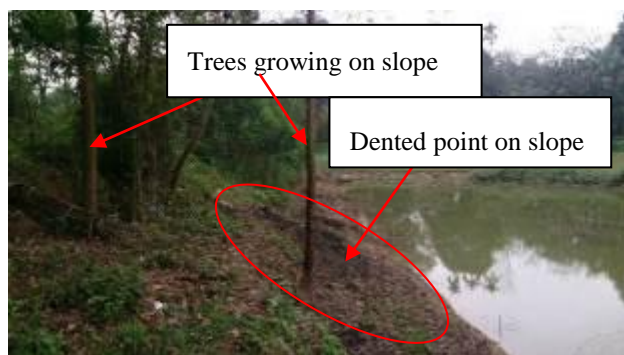
Current status of upstream slope of dam B
