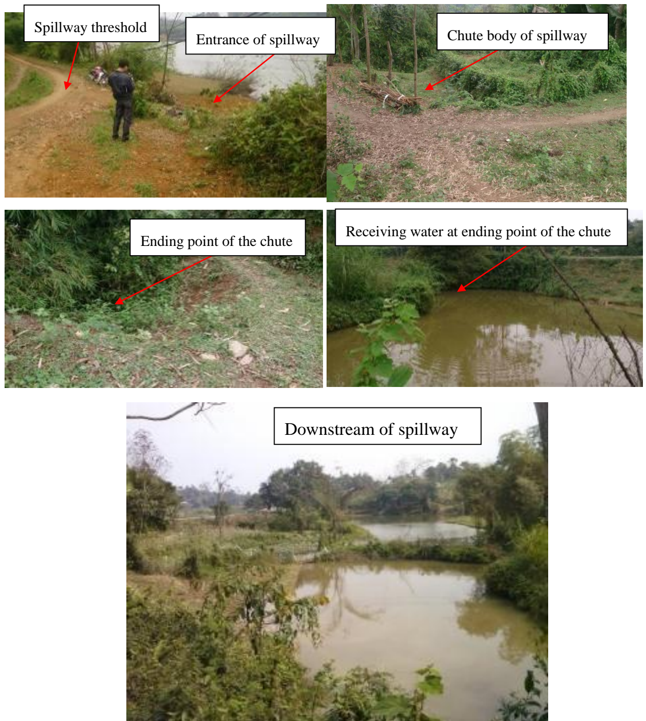
Figure 6 - 4: Condition of flood spillway
