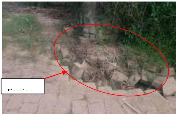
Figure 5-5: Bottom of the inlet in front of the sill of flood spillway is eroded
