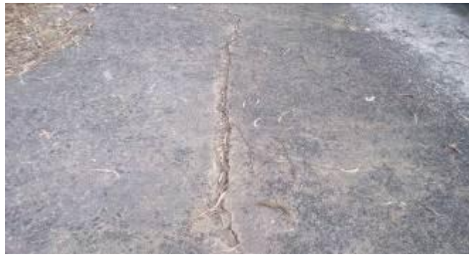
Figure 5-7: Bottom of narrow section has cracks
