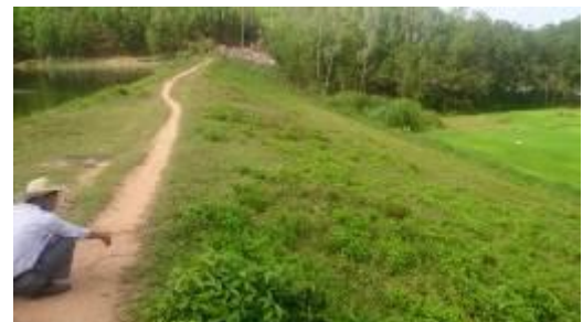
Figure 5-3: Dam slope is convex and concave in many places
