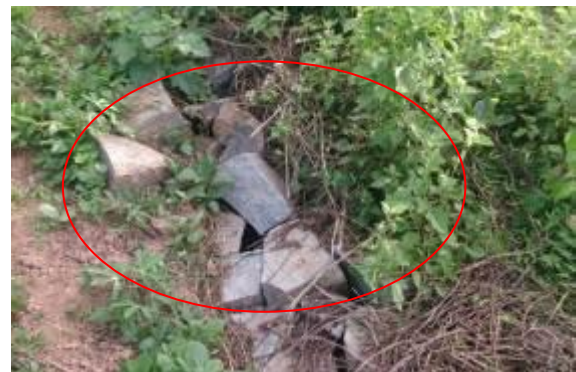
Figure 5-4: Stones for paving the downstream slope are displaced, and large gaps exist.
