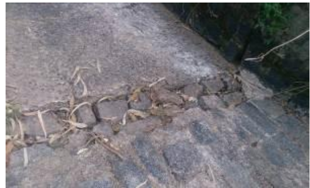
Figure 5-6: Ashlar stones in the sill bottom are eroded
