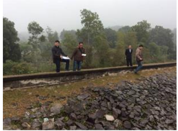
Figure 2.5: Broken cover of dam side
