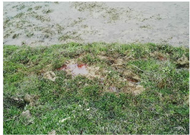
Figure 2.7: Seepage at downstream step of dam
