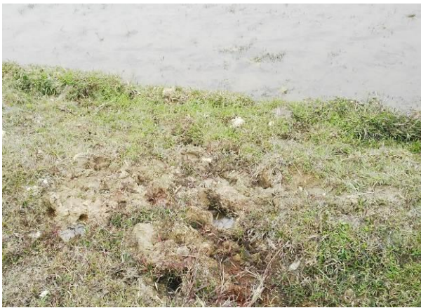
Figure 2.6: Seepage at downstream side of dam
