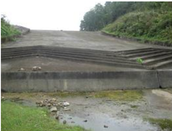
Figure 2.8: Seepage through body of spillway
