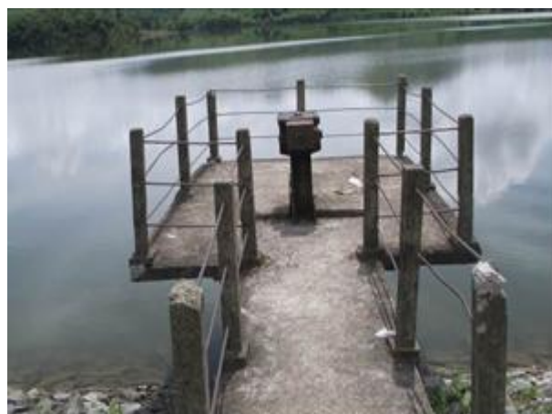
Figure 2.11: Manually controlled valve
