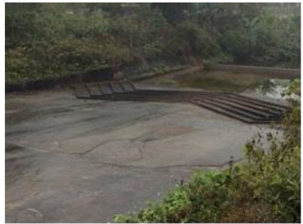
Figure 2.9: Erosion in cover of spillway with exposed reinforced steel
