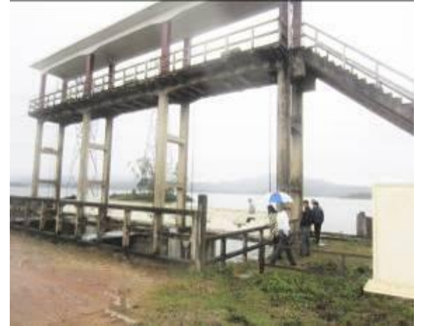
Phu Vinh reservoir field survey
