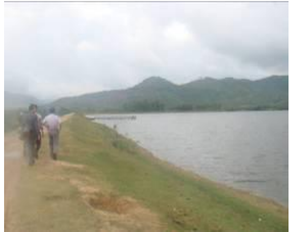
Thach Ban reservoir field survey.
