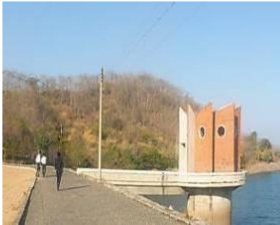
River Quao reservoir field survey
