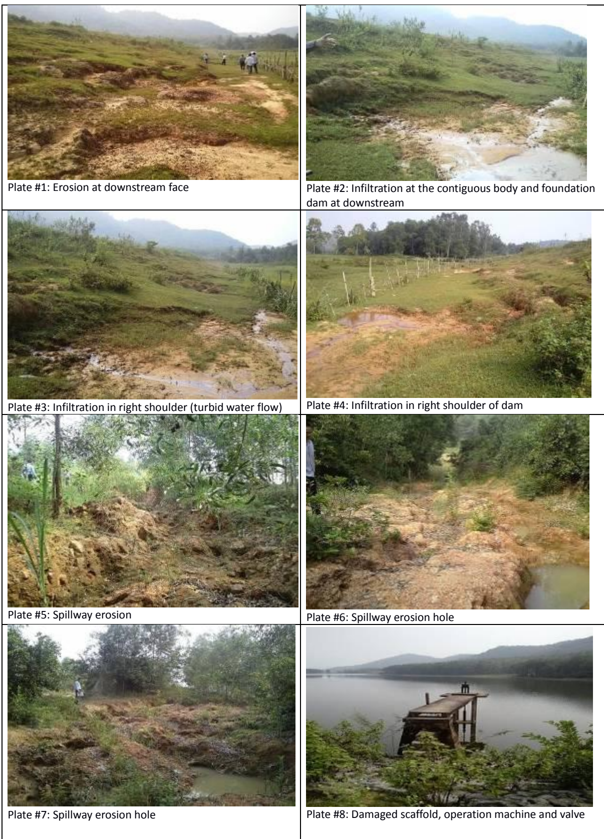
Figure 2.3. Photos showing the existing conditions of the dam and facilities
