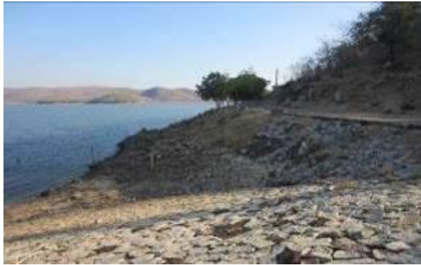
Figure 2.6: Peeled pavestone of the subdam upstream slope
