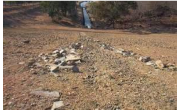
Figure 2.7: Subdam downstream slope eroded by rain
