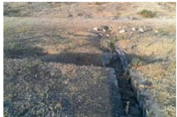
Figure 2.9: Damanged drainage ditch (subdam downstream slope)
