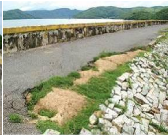
Figure 2.3 Subsidence of the main dam - Song Quao Reservoir
