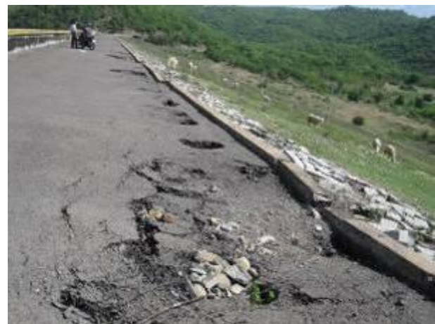
Figure 2.5: Peeled surface of the main dam - Song Quao Reservoir
