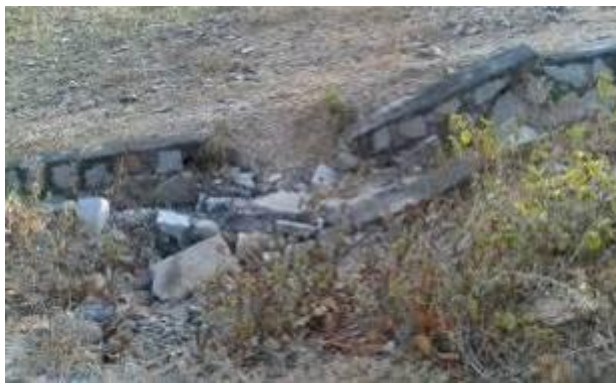
Figure 2.8: Subdam downstream slope subsiding and sagging
