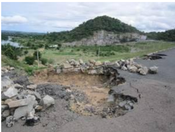
Figure 2.4: Seriously damaged surface of the main dam - Song Quao Reservoir
