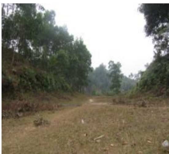
Figure 2-6: Entry of weir
