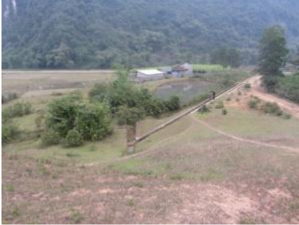
Image 1: The pathway leading to the dam viewed from the top of the dam
