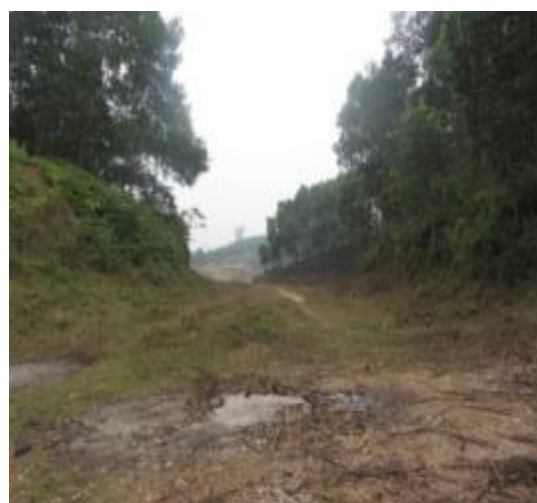
Figure 2-7: Damages caused by the overflow
