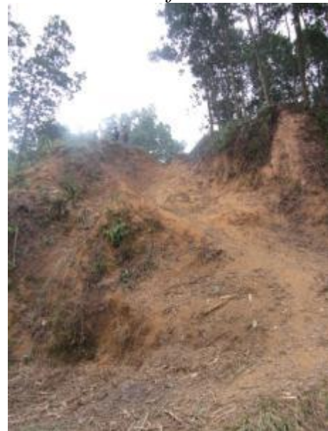
Image 12: Discharge through the overflow drain
