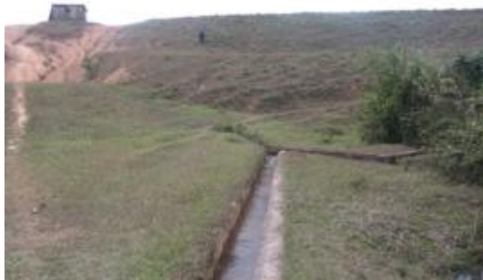
Figure 2-8: Tower of water intake
