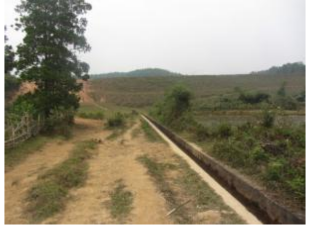
Image 2: Pathway leading to the top of the dam
