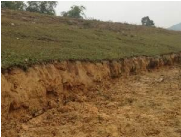
Figure 2 - 5: Sliding in the upstream slope of the dam
