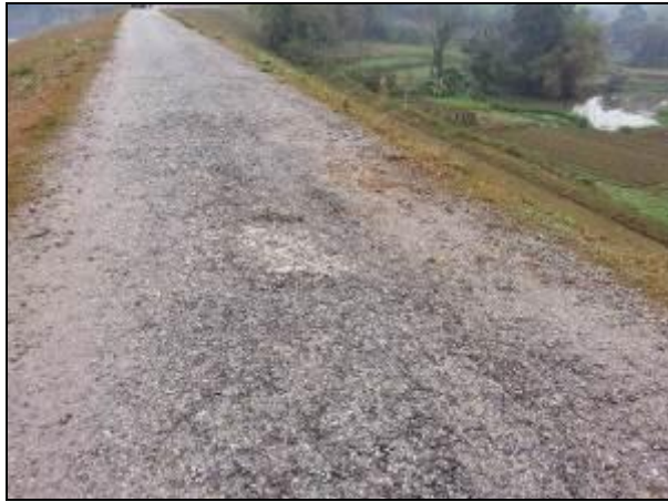
Figure 2 - 3: The crest of the dam is peeling from the middle view
