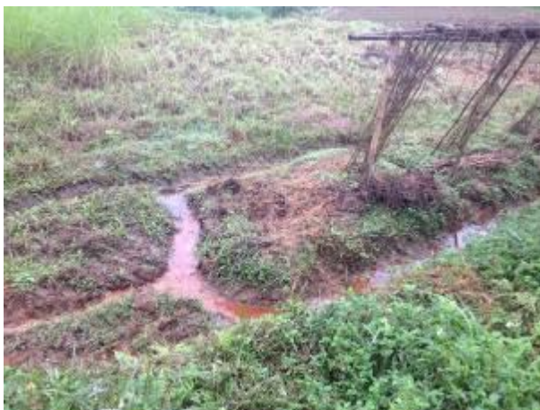
Figure 2 - 7: Infiltration in the downstream of the dam
