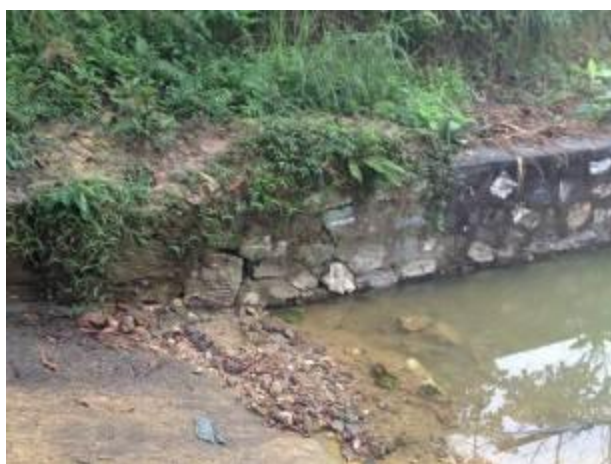
Figure 6 - 4: Side wall is damaged
