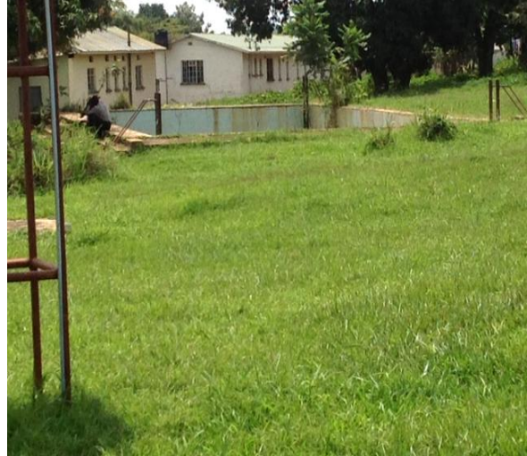
Photo 10: Old structures like these at Bukalasa ATC may have to be demolished to create room for new ones
