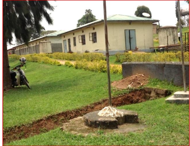
Photo 14: Such old buildings at UTC Bushenyi are historical and a treasure. A few of them should be preserved since they are still very strong
