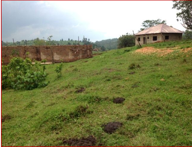
Photo 13: A semi-detached house (left) and a two bed-roomed house under construction for staff at UTC Bushenyi as a mitigation measure
