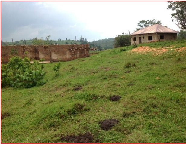
Photo 12: Staff houses under construction at UTC Bushenyi
