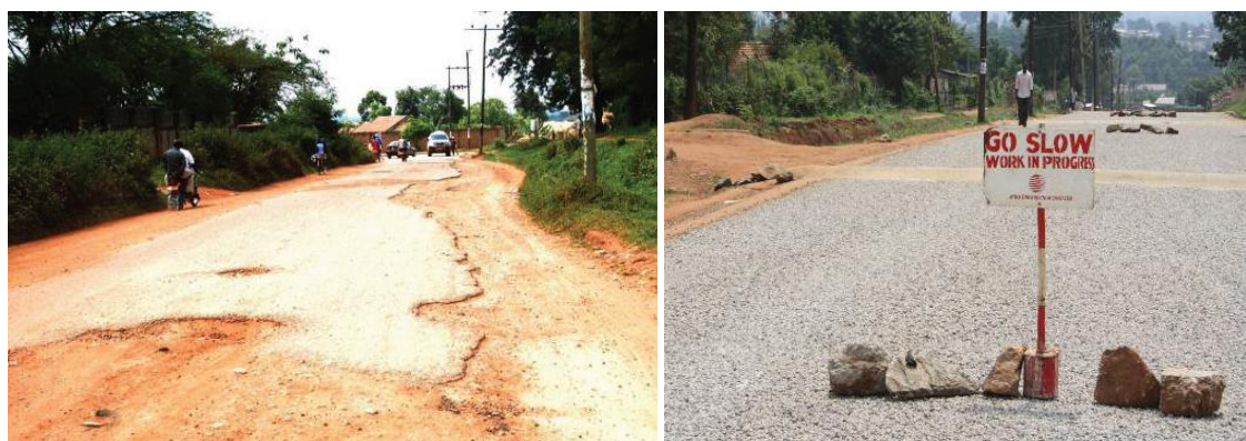
Photo 3: Kakungulu Drive in Mbale before and during rehabilitation
