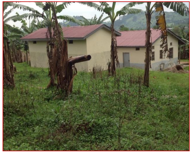
Photo 10: Old staff houses at UTC Bushenyi
