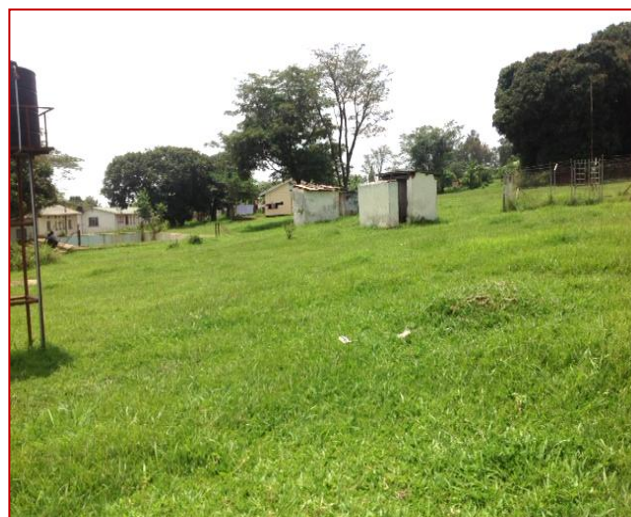
Photo 4: Dilapidated structures at Bukalasa Agricultural training College.
