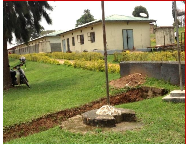
Photo 13: Old but relatively good-condition staff houses at UTC Bushenyi
