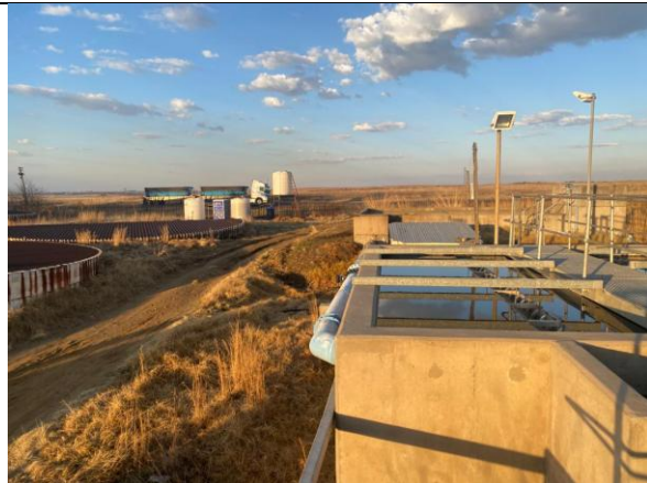
Water treatment plant to be upgraded and old reservoirs to be decommissioned
