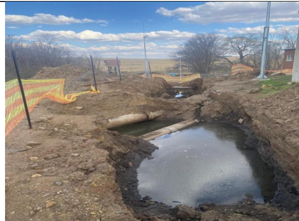
Asbestos pipes to be replaced with uPVC pipes
