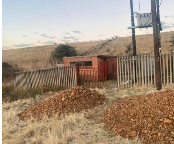
Intake for pump repairs and line refurbishment
