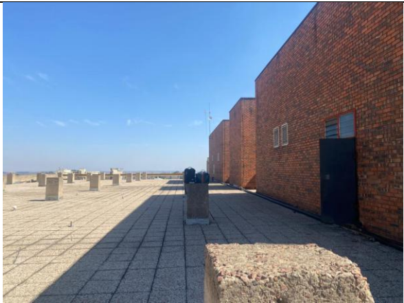
Office Building Rooftop for solar panels
