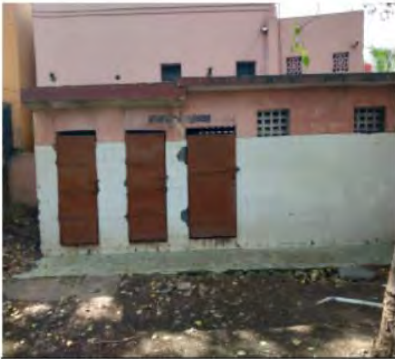
Proposed location for toilets to be repaired
