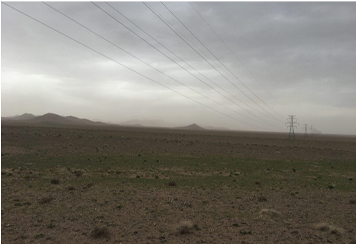
Figure 3: Photo of Pol-e-Hashimi substation land
