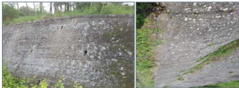
Figure 2-21_Retaining wall in good conditions - Golem
