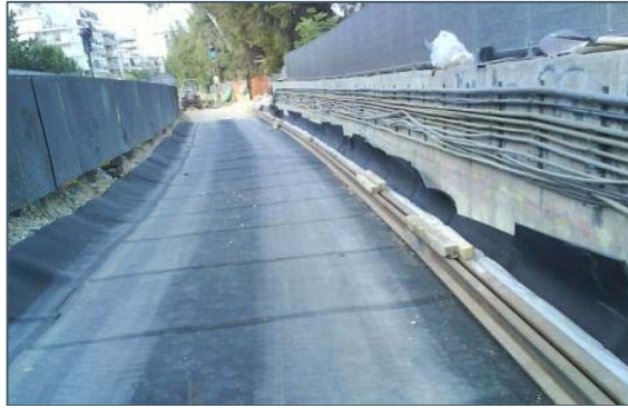
Figure 6-12_Ballast mat application (before laying ballast)
