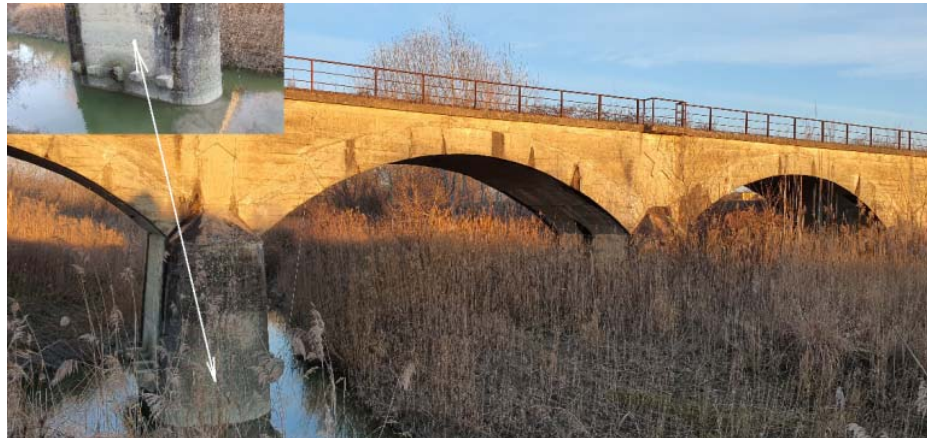
Figure 5-19_Darsi River Bridge (km 23+150)
