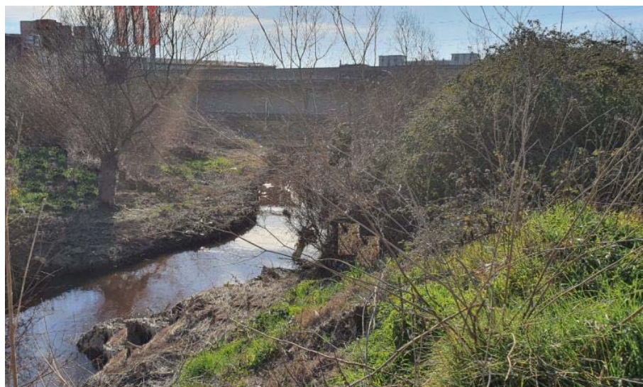
Figure 5-18_ Lishati River Bridge (km 15+420)
