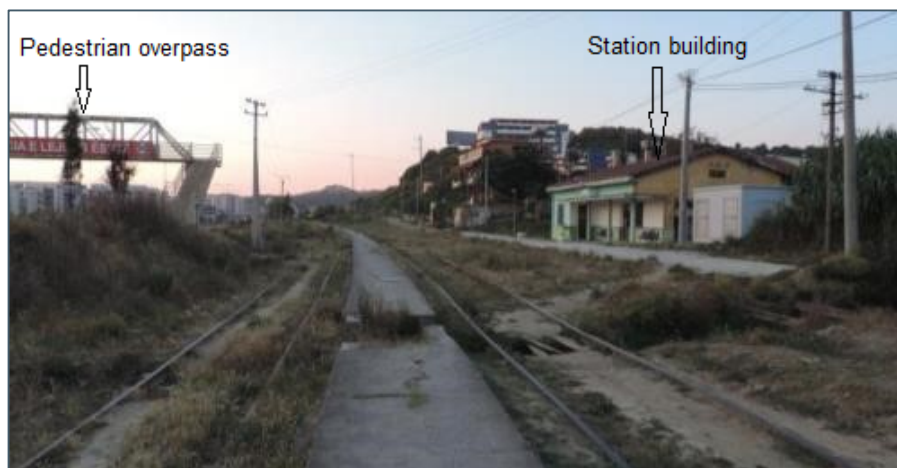
Figure 2-19_Pedestrian overpass that serves only the motorway – Golem station
