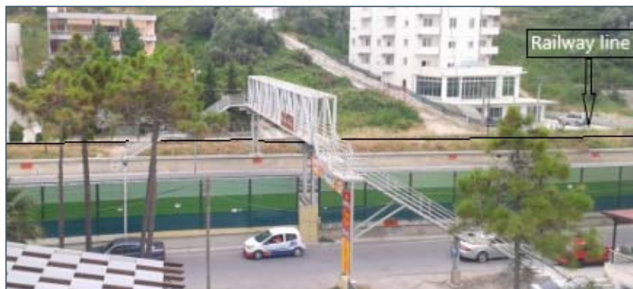
Figure 2-20_Pedestrian overpass (Km 7+360) serving only for the motorway
