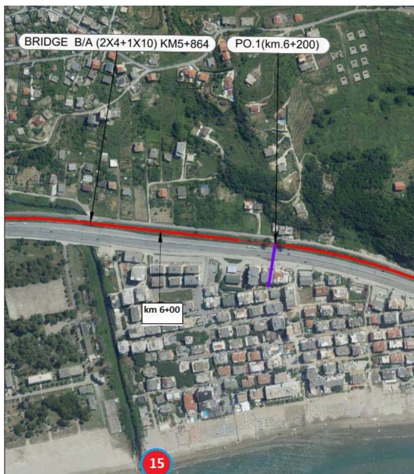
Figure 5-23_Drainage channel discharging into the sea at Km 5+864
