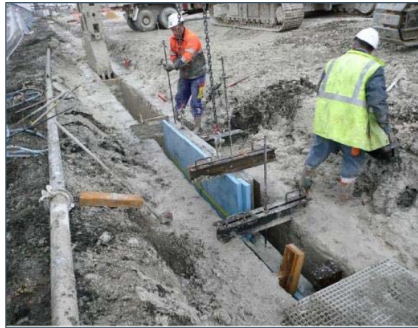
Figure 6-13_Excavation and filling of near track trench
