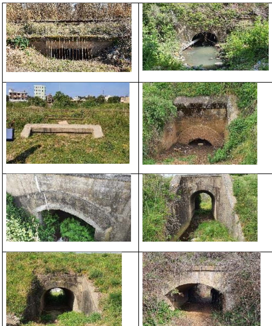
Figure 2-25_Existing situation of the majority of the railway line culverts
