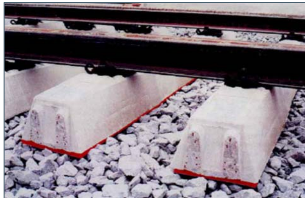
Figure 6-11_Under sleeper pads
