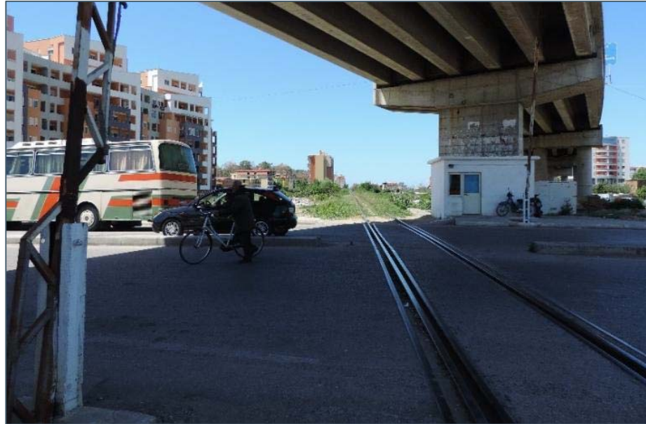
Figure 2-18_Motor road overpassing the railway line at km 5+180
