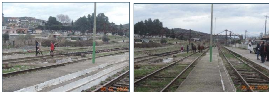
Figure 2-36_ Unauthorized pedestrians and animals crossing at Rogozhine station area
