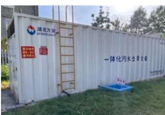
Fig 12: Rural WWTF (80t/d) operated by a third party, Honghu, Hubei
