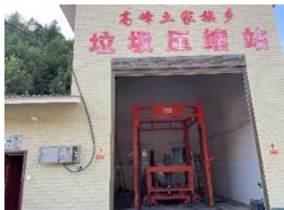
Fig 19: Township solid waste transfer station (compacting facilities, leachate collection tank), Cili, Hubei
