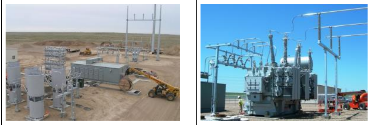
Figure 2-6: Typical Collector Substation
