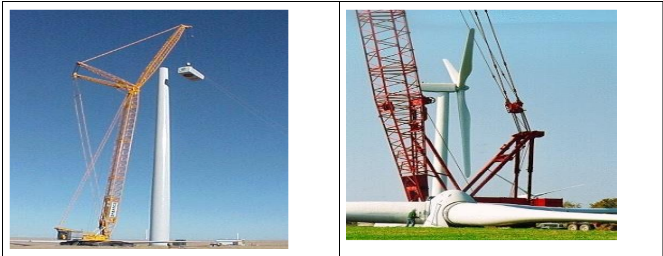
Figure 2-5: Typical Tower erection
