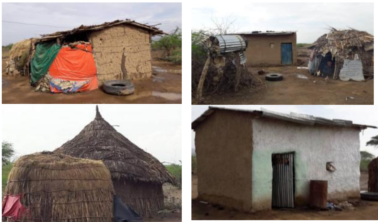
Photo 02: Typical Affected Houses by Type of Roofing
