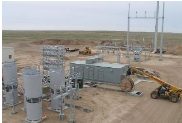
Typical Collector Substation
