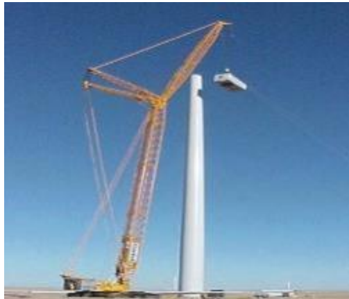
Typical Tower erection
