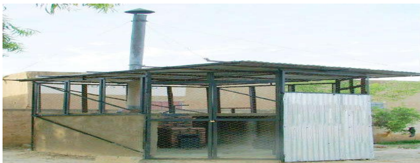
A De-Montfort Waste Disposal Unit
