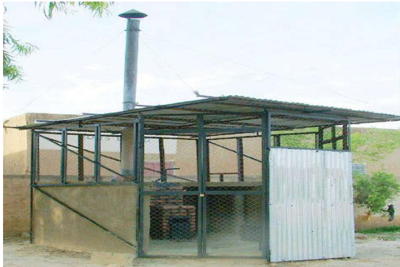
Figure 3.0: A De-Montfort Waste Disposal Unit
