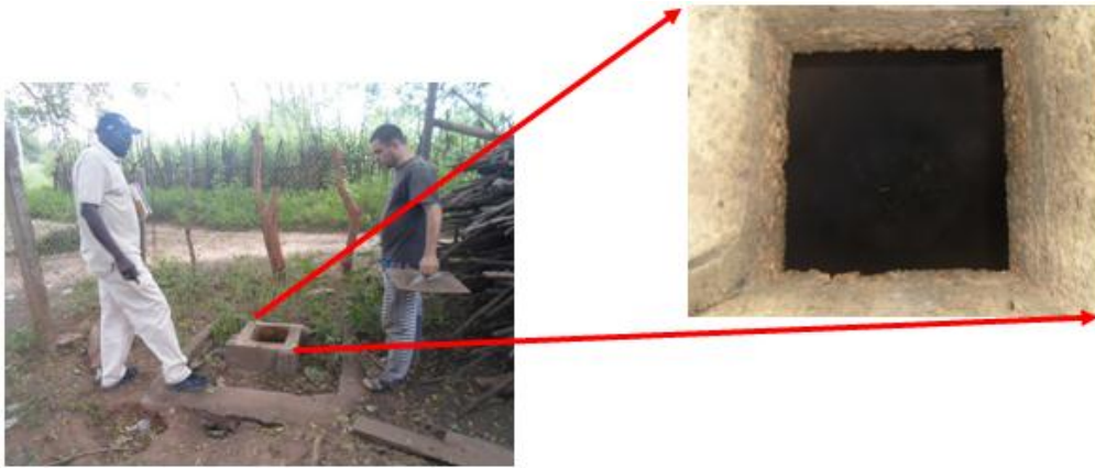
Figure 62 Concrete lined pit for sharps disposal at a Clinic
