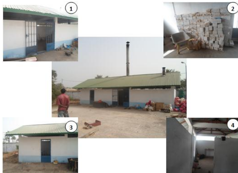
Figure 42 Kotu - Temporary storage Area attached to incinerator. 1...Main entrance to the incinerator. 2...Stacked Sharp Boxes in the Temporary storage area. 3...Entrance to the Temporary Storage area. 4...Inside the Temporary Storage Area.
