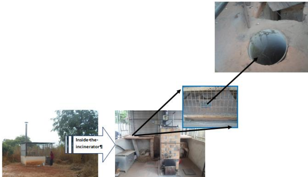
Figure 64 Pathological Waste pit at Incinerator sites
