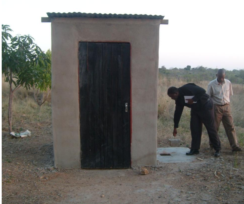
Pit with Pit Latrine for home based care
