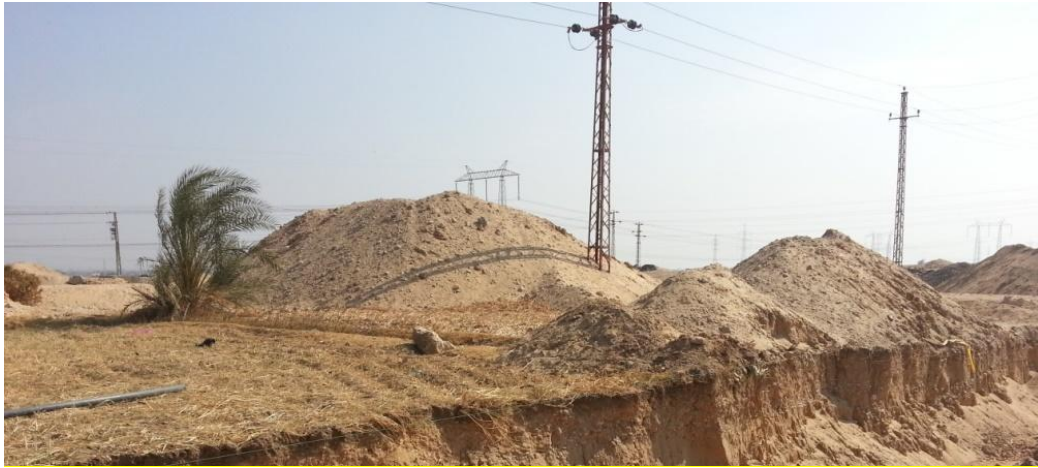
Figure 2-5: Site of the New PRS in Gerga
