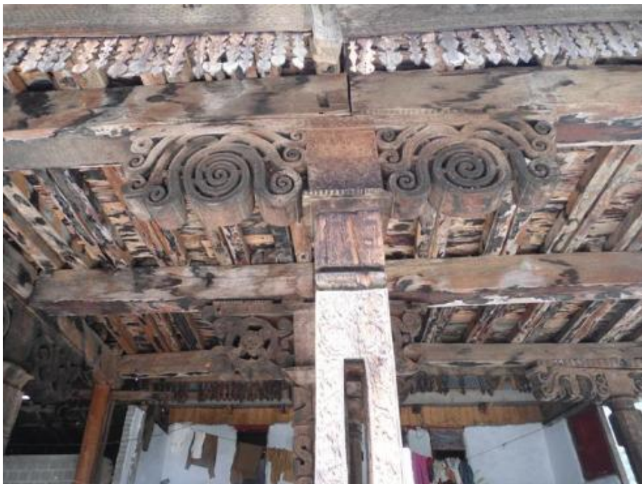
Figure 5.9: Seo Mosque showing Wooden Pillar and Brackets
