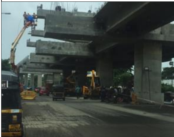
Ongoing work with unsafe conditions (safety hazard) with moving traffic on Road
