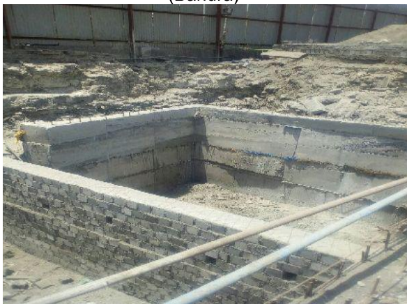
Sedimentation Tank construction at Batching Plant (Bandra)
