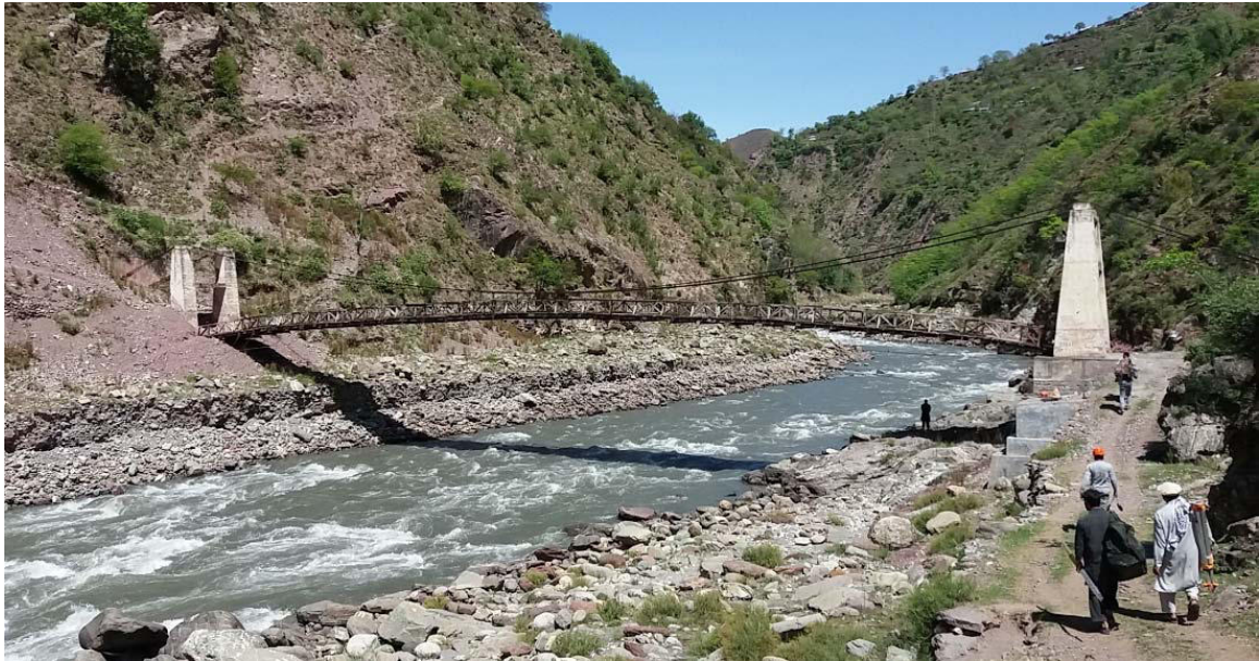
Close up of bridge near cross sections at EF Site 2
