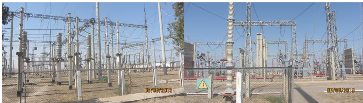
Photograph 3. Switchgears 110 KV and 220 kV
