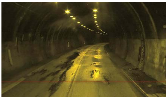
M17 Tunnel Crnaja km 15+082
