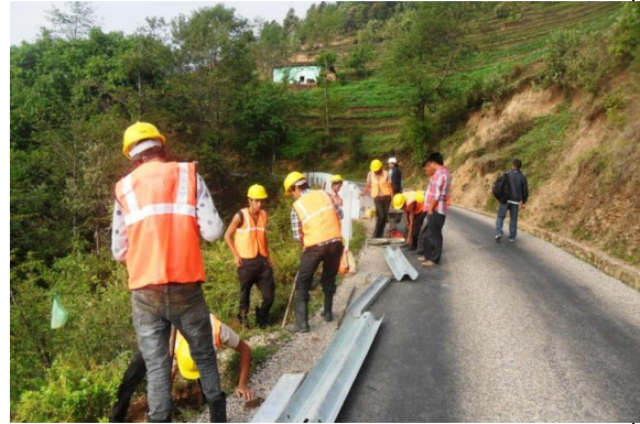
Steel W-Beam Crash Barrier under installation at chainage 2+300.00 of Khodpe-Bajhang Road
