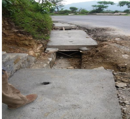
Improvement of road side drain to make the road safer in Road Safety Pilot Project, Pokhara
