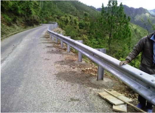
M20 Concrete work for fixing channel post of Steel W-Beam Crash Barrier at chainage 2+220.00 of Khodpe-Bajhang Road
