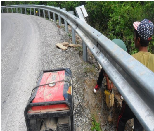
Application of Rock Breaker for proper installation of Steel W-Beam Crash Barrier at chainage 16+760.00 of Khodpe-Bajhang Road
