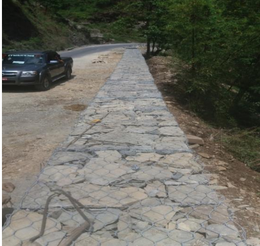
Installation of Gabion Barrier on Siddhartha Highway
