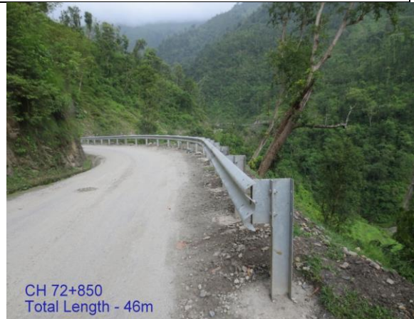
Steel W-Beam Crash Barrier under installation at chainage 72+850 Tallodungeshore Jumla Road
