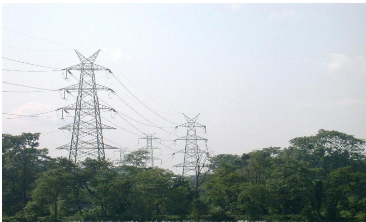
Image 1a: Actual 400 kV Transmission Line (1)
