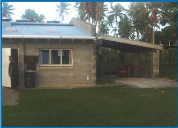
Photo 1: Existing Diesel Generation Station at Ha'afeva
