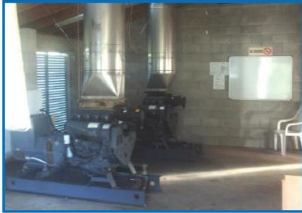
Photo 2: Existing Diesel Generators at Ha'afeva Power Plant
