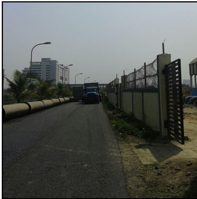
10. End of Transmission Line at BS-1
