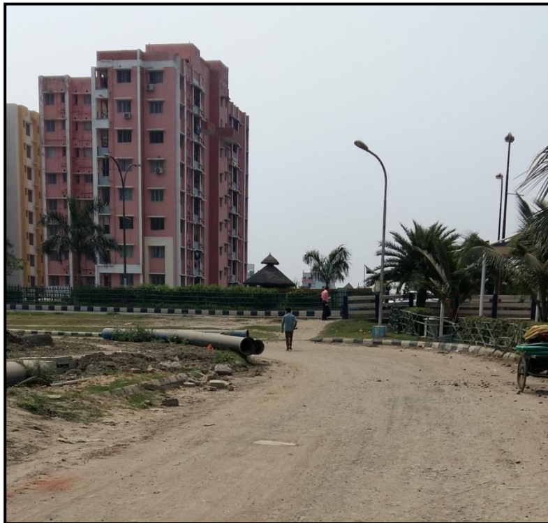
8. Location for Micro-tunneling Pit near bridge
