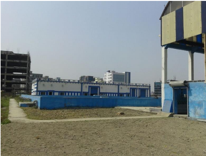
Site for proposed clear water sump and booster station
