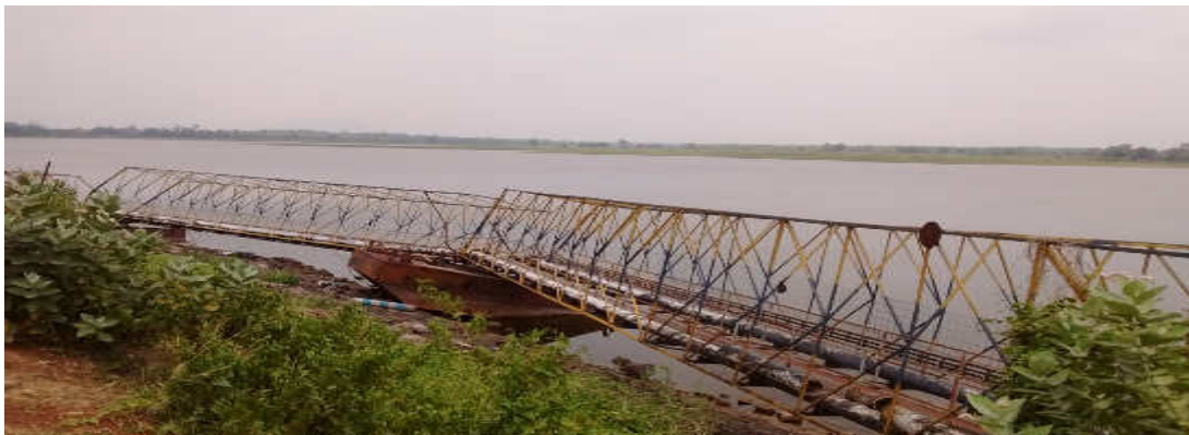
Sali reservoir and the raw water main
