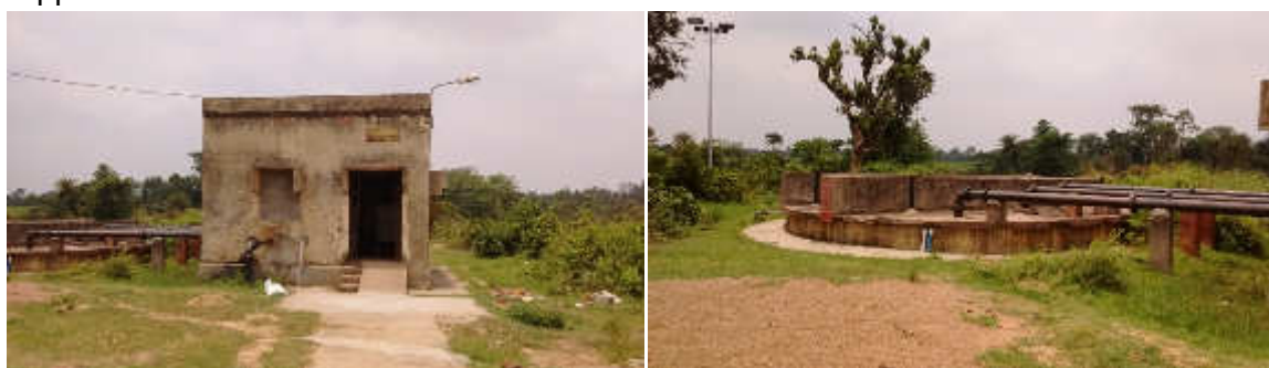
Pump House: Charadihi WS Scheme and the CWR
