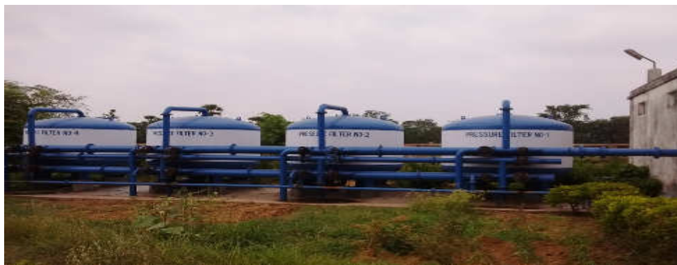
Pressure Filters at the Gangajalghati WTP
