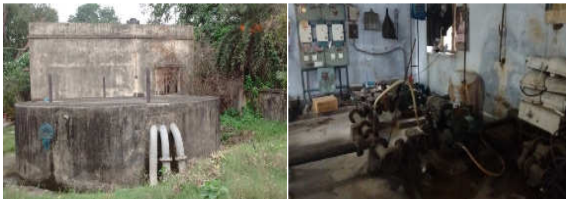
Existing ground level reservoir and pump house
