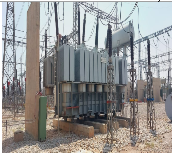
A view of 250 MV of 220/132kV at T-7
