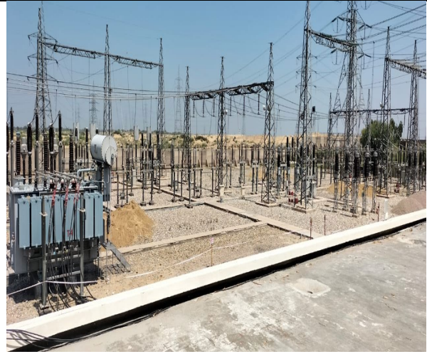
132kV Switchyard of the G/S
