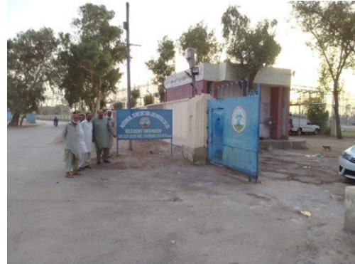
A view of the G/S from the entrance – access road
