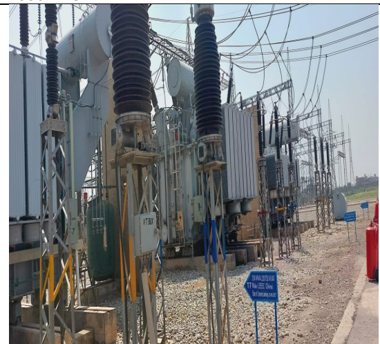
A view of 250 MV of 220/132kV at T-7
