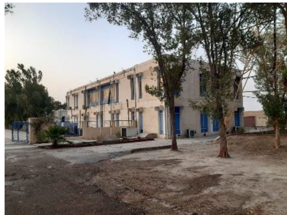
Main Office Building at the GS
