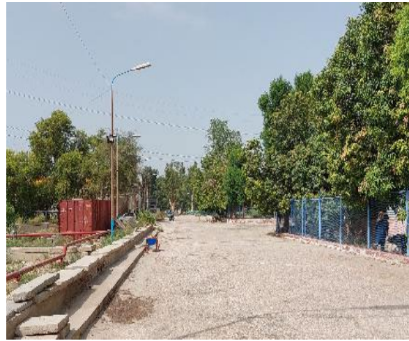
Entrance of Main office Access Road Guddu Barrage Road
