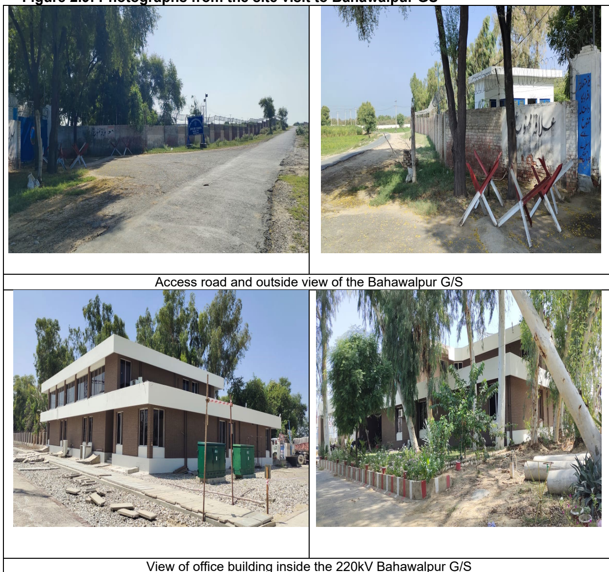
Figure 2.9: Photographs from the site visit to Bahawalpur GS
