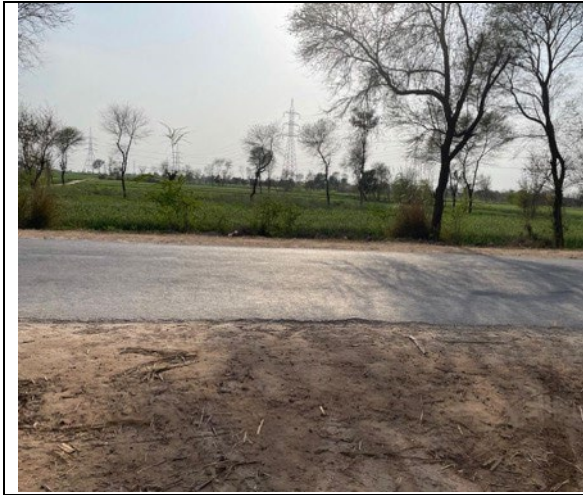
View of the front site towards Painsra – Bhawana road of 500 kV, 220kV & 132kV Grid Station (Faisalabad West)
