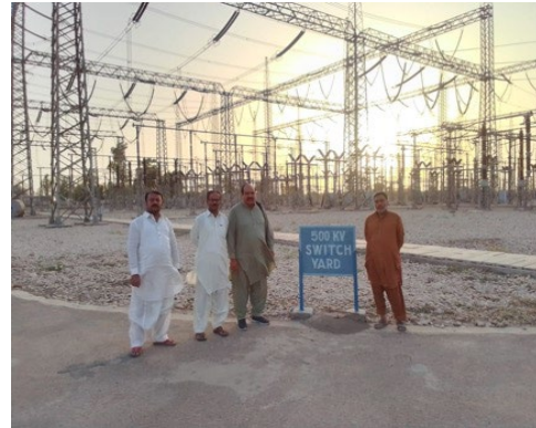
View of 500 kV switchyard
