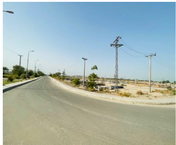
Open area along with the entrance road to switchyard is visible inside the G/S
