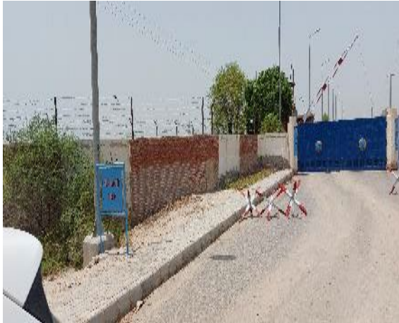
Entrance and access road to Rahimyar Khan GS
