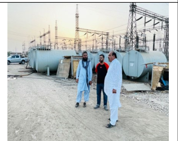
Visiting the switchyard with the TM and contractor
