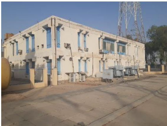
Main Office Building at the GS
