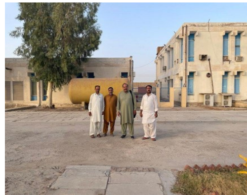
View in the front of office buildings
