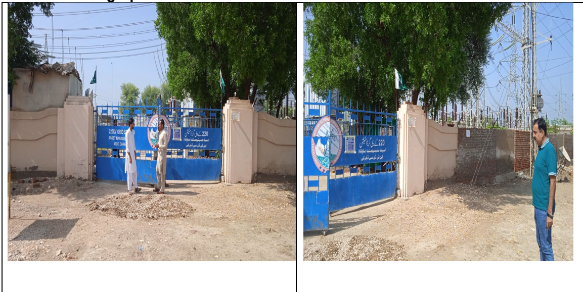
Access road and main entrance of 220kV Daharki Grid Station
