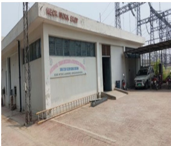
Technical Building at GS
