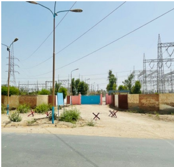
Another View of main entrance from Main Guddu Barrage Road
