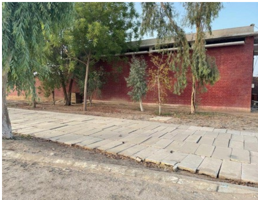
Workshop building of G/S
