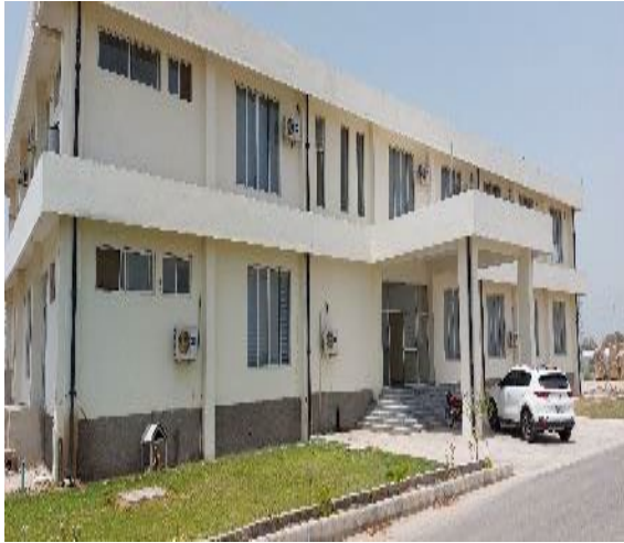
Main Office Building at GS
