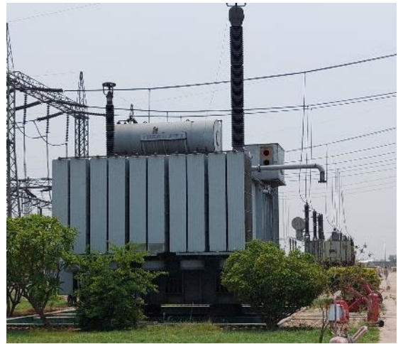
A Spare 220 kV Transformer at the EGS
