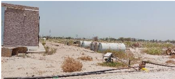
Transformer Oil Tanks Placed at Unsealed Surface without Secondary Containment
