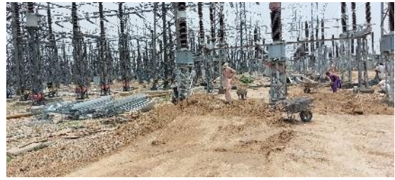
Under-construction Switchyard at the EGS. Men at work without PPE
