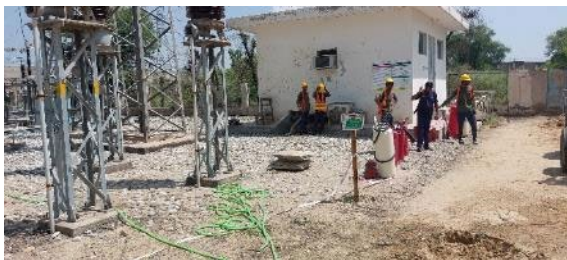
Empty Drums of Transformer Oil on Unpaved Surface. Residual Oil can be Seen in a Bowl
