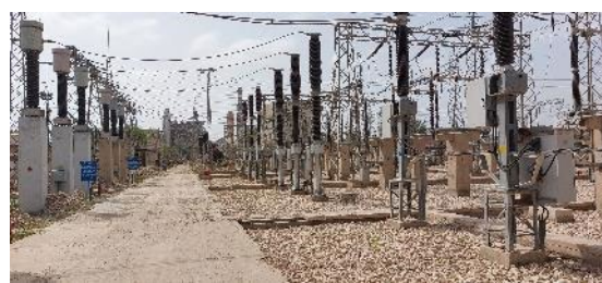
220 kV Switchyard at the EGS
