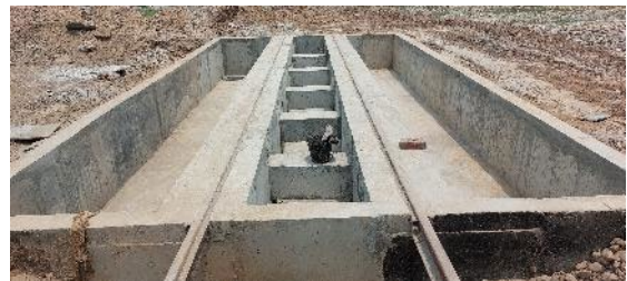
Under-construction New Bays for new Transformer
