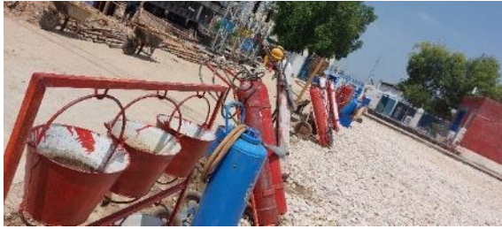
Firefighting Equipment. Buckets were found with Rainwater
