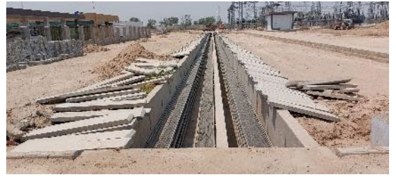
Under Construction Cable Line Trenches
