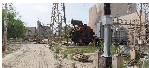
Abandoned and Burnt Transformer Kept on Unsealed Surface
