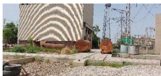
Rusted Transformer Oil Tanks on Unsealed Surface
