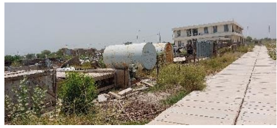
Transformer Oil Tanks Placed at Unsealed Surface without Secondary Containment
