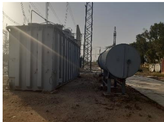
Transformer without Secondary Containment
