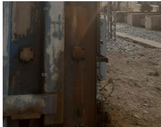
Leakage from a Transformer
