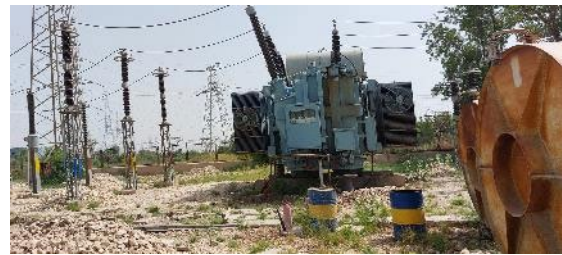
Transformer and Oil Tank on Unsealed Surface
