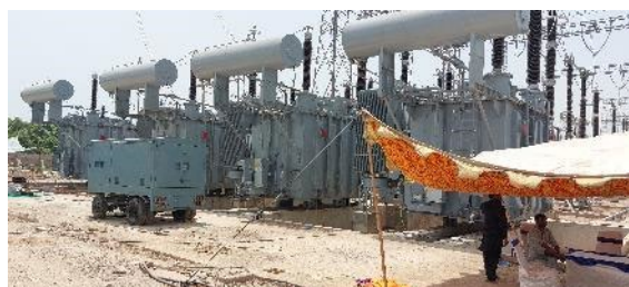
Abandoned Transformer Placed at Unsealed Surface near Transformer Bay
