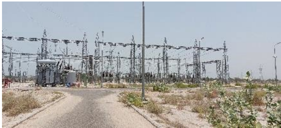
Spare Transformer at Unsealed Surface near Switchyard Premises
