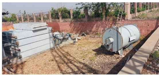
Transformer Oil Tanks on the Unsealed Ground
