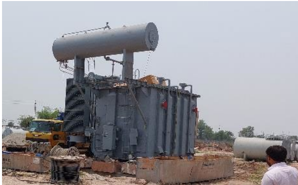
A Spare Transformer Kept on Unsealed Surface
