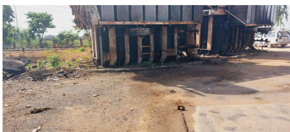
Transformer Oil Spilled Stains on the Grounds
