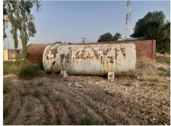
Rusted Transformer Oil Tanks Kept on Unsealed Surface
