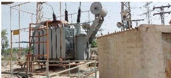
Transformer Kept on Unsealed Surface
