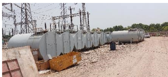
Transformer Oil Tankers Placed at Unsealed Surface without Secondary Containment
