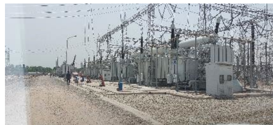
Under-construction New Bays for new Transformer
