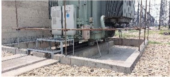
Secondary Containment for Existing Transformers
