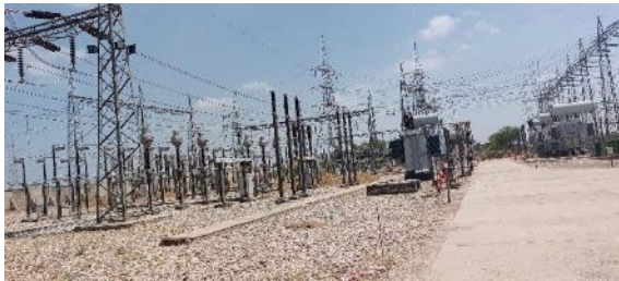
220 kV Switch Yard at EGS
