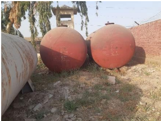
Transformer Oil Tanks kept on Unsealed Surface
