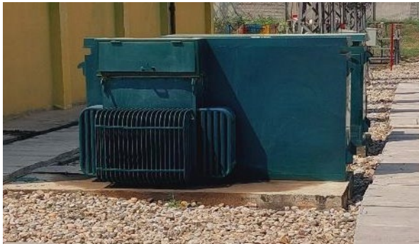
Oil Stains at Base of Auxiliary Transformer at EGS
