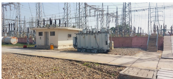
Spare Transformer on the Unsealed Ground
