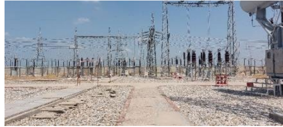
132 kV Switch Yard at EGS
