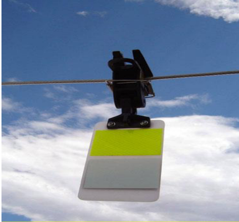
Figure 46 firefly bird flapper/diverter recommended (or equivalent) for this transmission line (Birdbusters, 2017)
