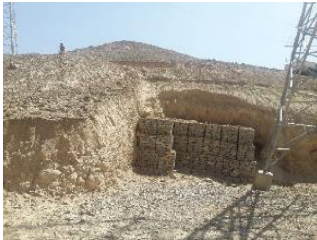
Figure 39 Soil erosion protection retaining wall currently used for tower foundation at Arghandeh
