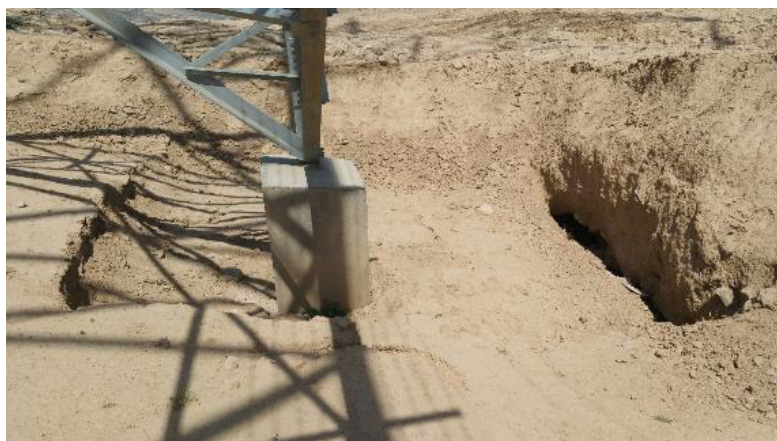
Figure 40 Example of poorly compacted soil in tower foundation in the Arghandeh area
