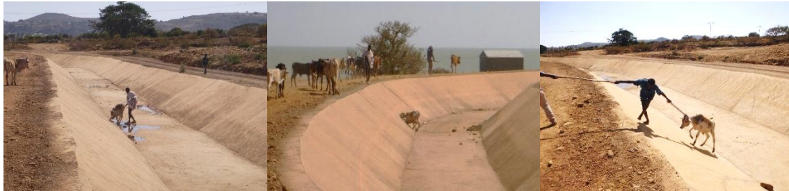
Figure 65 Stuck cow in a lined canal
