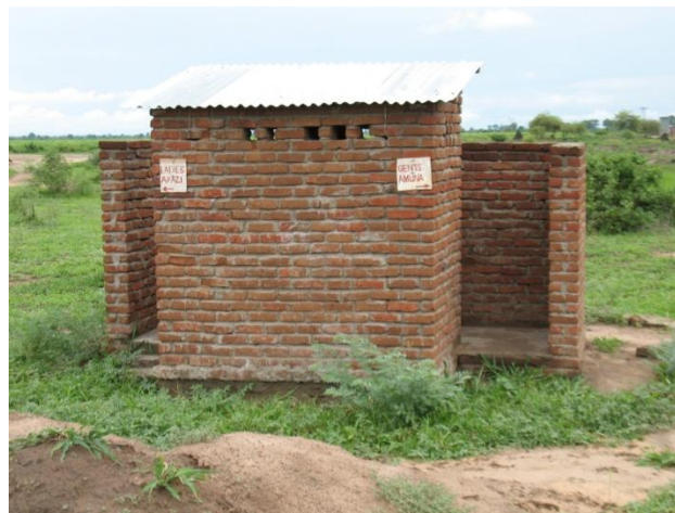
Figure 69 Communal pit latrine in Kasinthula, an elegant but rarely used structure
