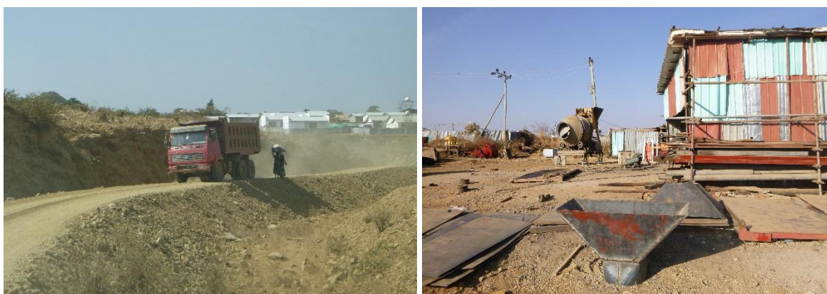
Figure 66 Trucks and pedestrians sharing construction roads &amp; rubbish in construction camps
