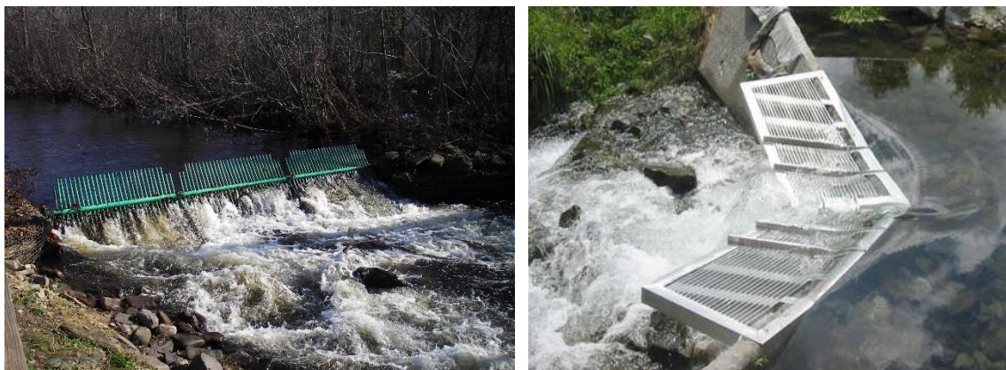
Figure 91 Examples of fish weir and rack
