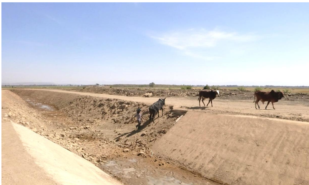
Figure 80 Earth offers better grip than concrete
