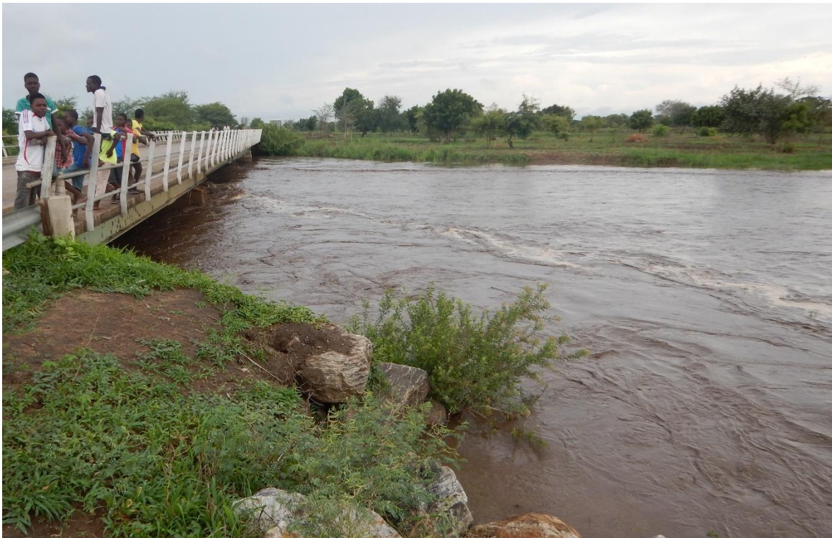
Figure 15 Mwanza River at the Bridge of the M1 National Road, completely overflowed the January 27th 2016
